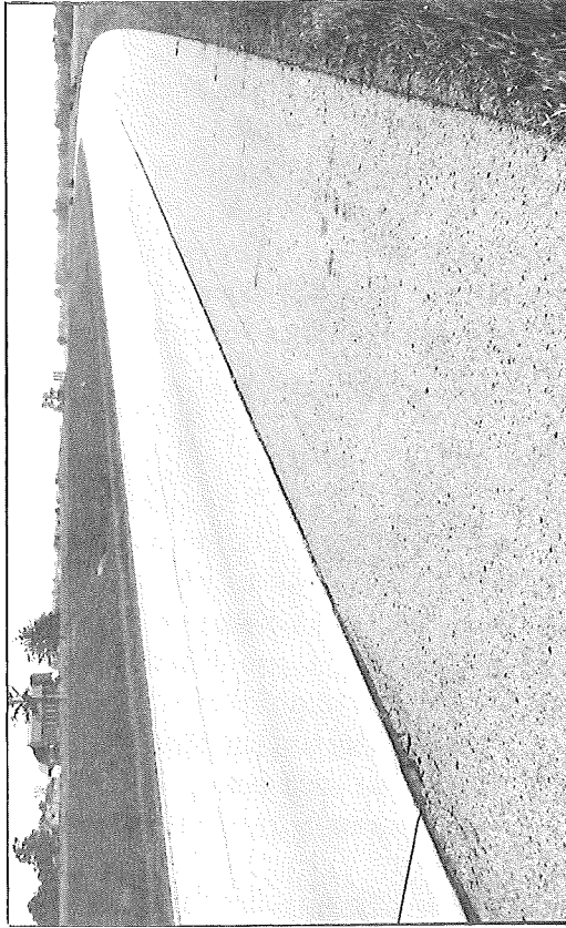
Full-depth bituminous base course and wearing course
