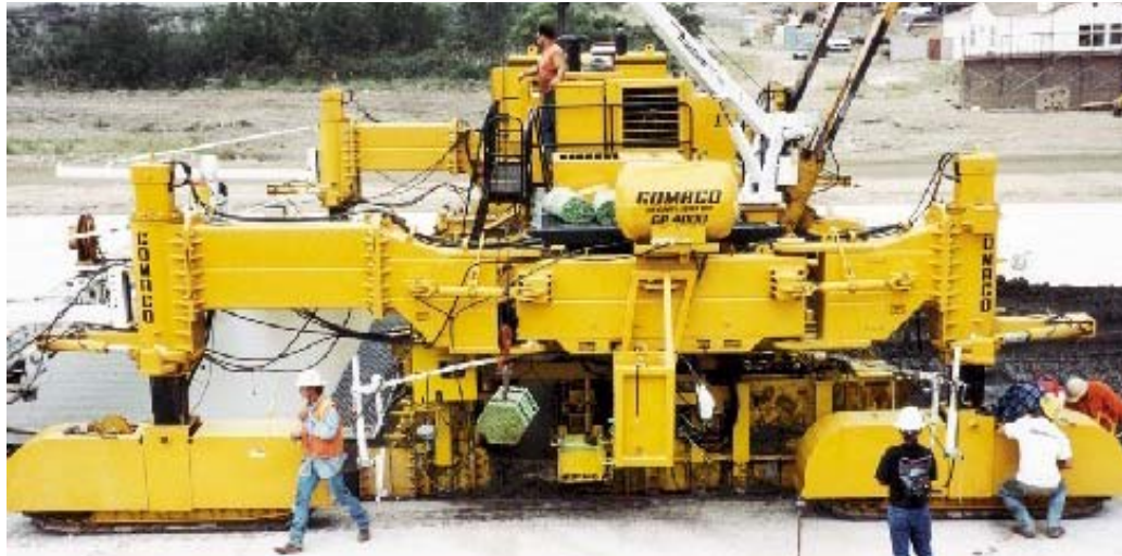
(a) Typical Slipform Paver with inbuilt Dowel Bar Inserter
