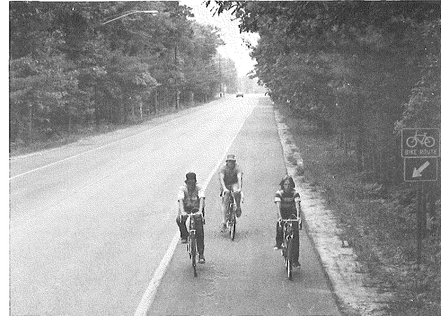
CLASS II – A restricted area for the exclusive or semi exclusive use of bicycles. Cross-flows by motorists, to gain access to driveways or parking facilities, is allowed. Pedestrian cross-flows, to gain access to parked vehicles, bus stops or associated land use are also allowed. Through travel by motor vehicles or pedestrians is generally not allowed. However, vehicle parking can occur adjacent to these bikeways.
