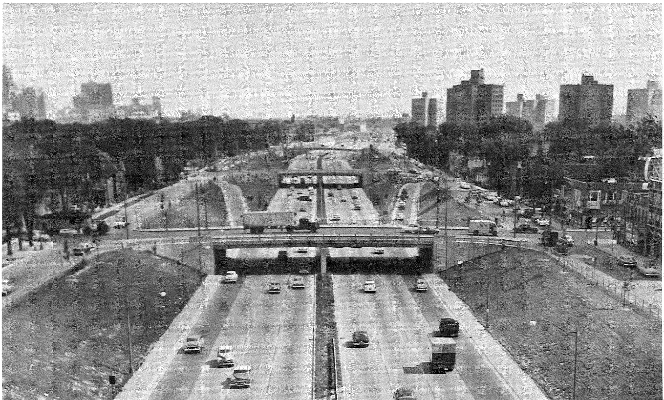
Expressway construction, such as this portion of the Lodge Expressway in Detroit, offers the most practical means of relieving congestion on some heavily traveled urban trunklines. Experience shows expressways move well over twice as many vehicles per lane as arterial surface streets, with three times the average speed and safety.
