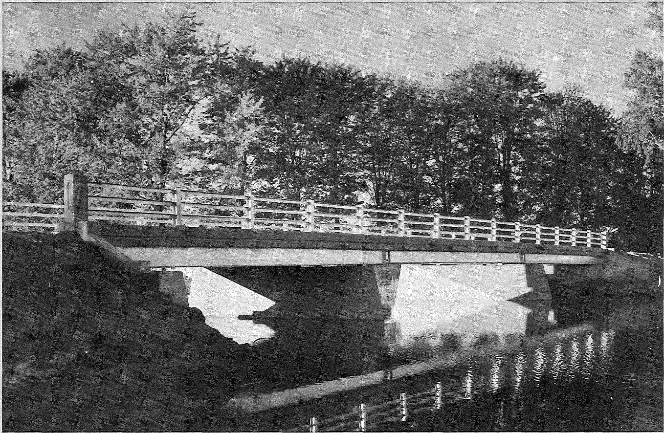
This recently constructed bridge over the Pine River in Arenac county meets county primary construction standards. The 20-year needs call for construction, or reconstruction of 1,523 bridges on the county primary system.
