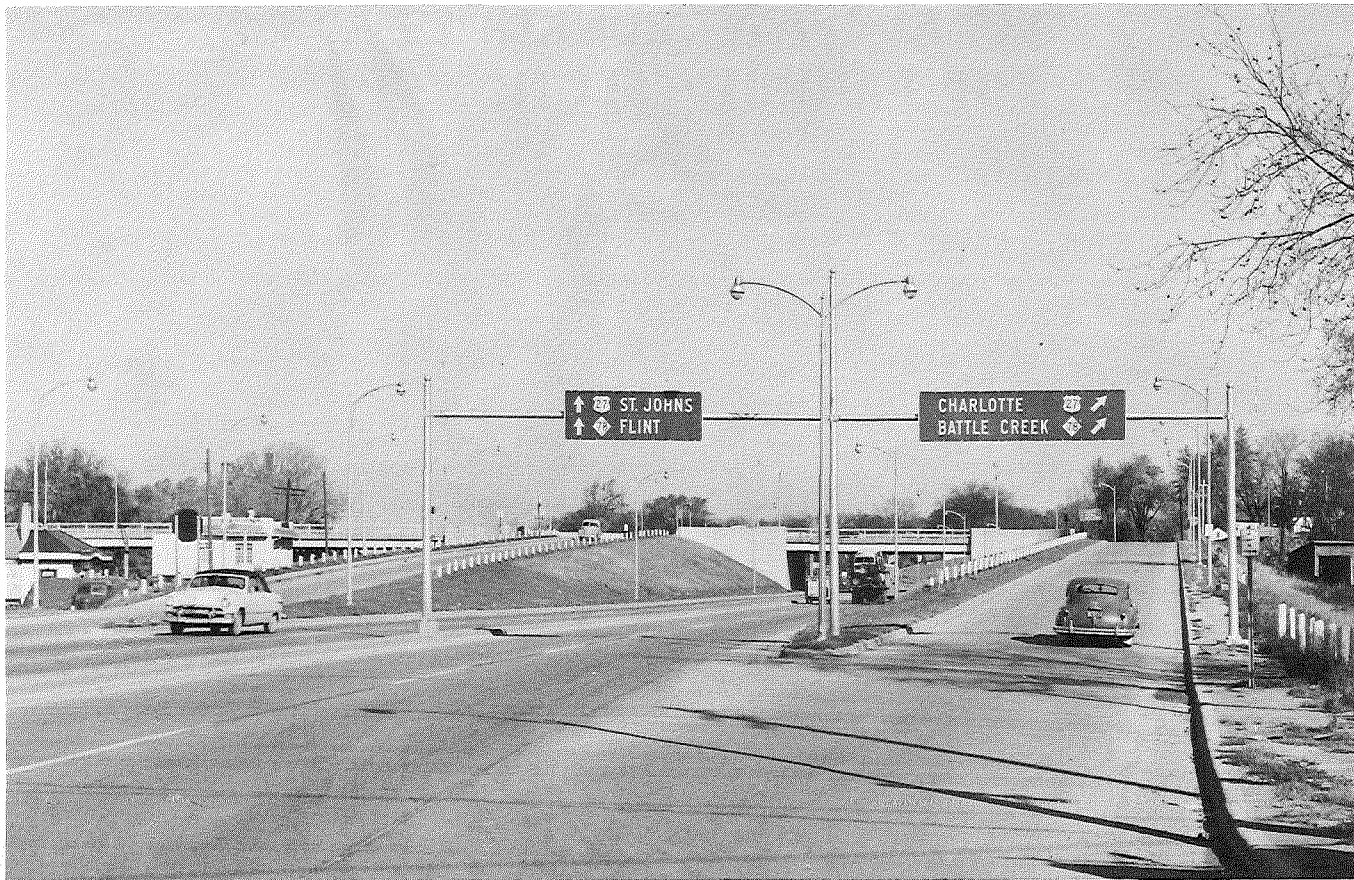
Increased efficiency results from proper signing and marking of routes. Overhead signs which can be seen from a distance, are particularly effective for travelers unfamiliar with an area.
