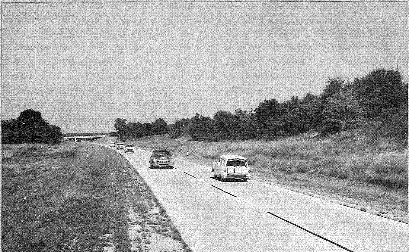
This is a portion of U.S. 12 near Kalamazoo which is being developed to Interstate System expressway standards by stage construction. Contracts for completion of this section as a four-lane divided facility with full control of access are presently scheduled for letting late this year.
