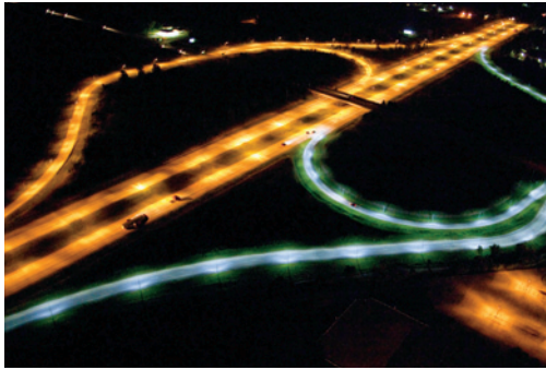
I-275/Eureka Road interchange, west of the Detroit/ Wayne County Metropolitan Airport. Shown at upper left are traditional high-pressure sodium lights (along mainline I-275 in both directions and the northbound ramps), with pilot LED lights shown in the lower right (along the southbound ramps).
