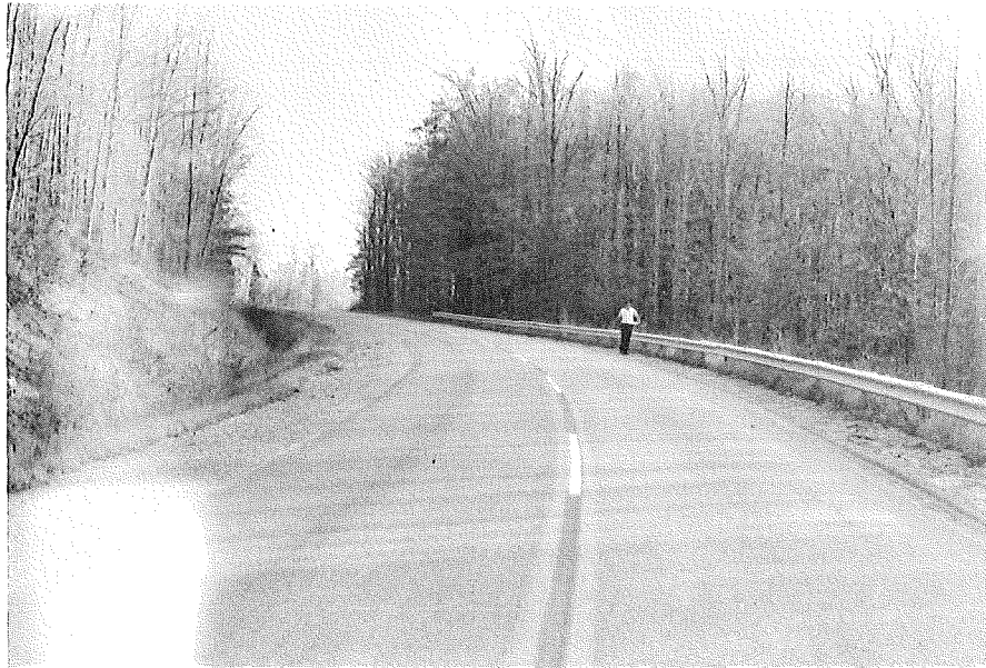
SOUTHBOUND CO. RD. 491
