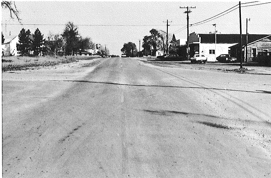
EASTBOUND CO. RD. 612
