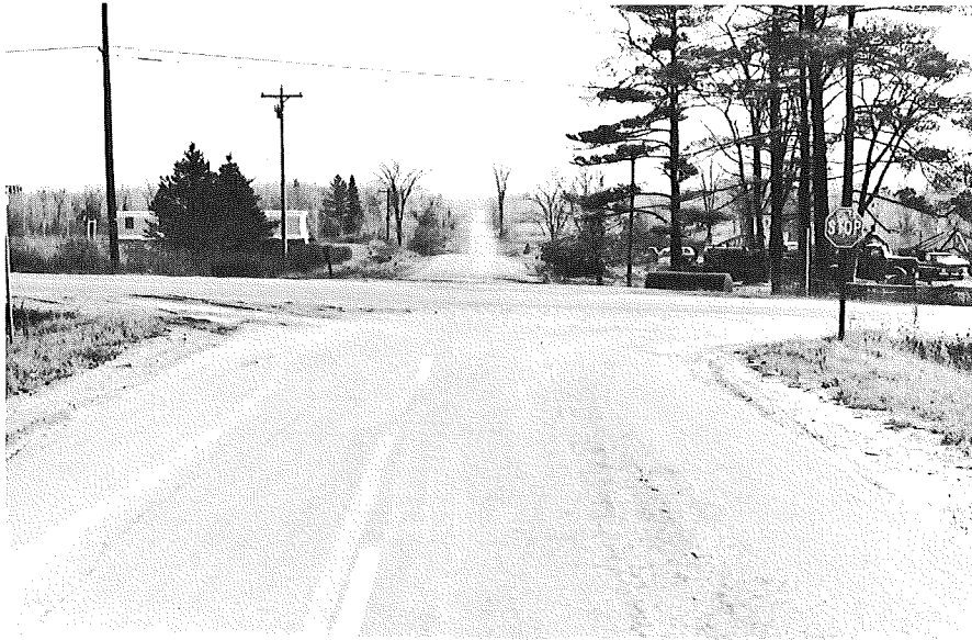
EASTBOUND CO. RD. 624
