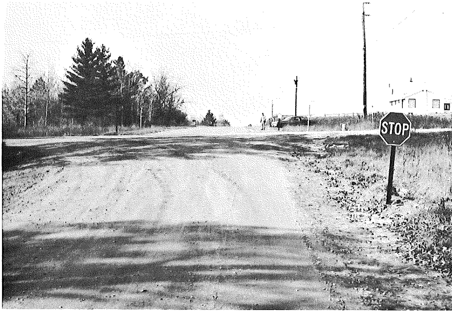
WESTBOUND CO. RD. 624
