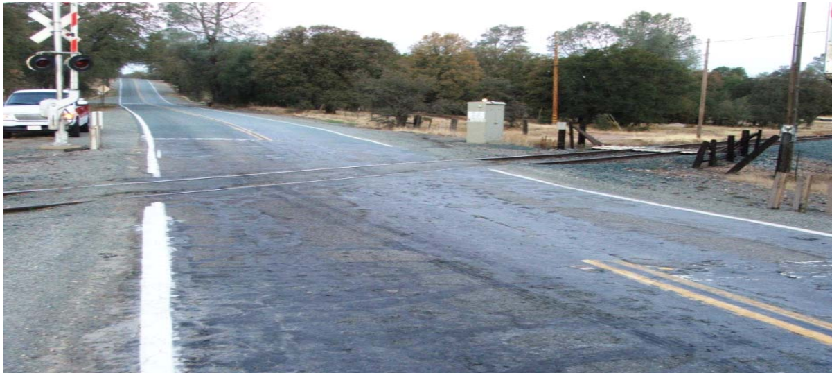
Figure 2 - Asphalt Crossing Surface
