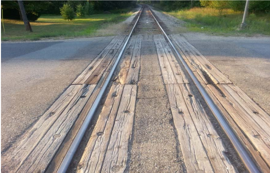
Figure 5 - Timber Crossing Surface
