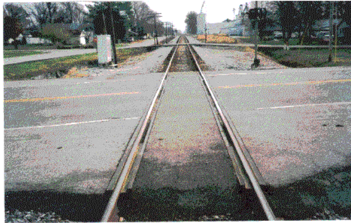
Figure 2.1f US 60 (Stanley) crossing with underlayment.
