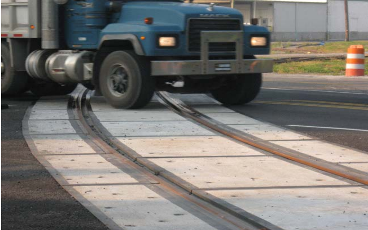
Figure 3 - Concrete Crossing Surface
