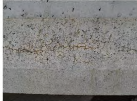
(b) Bottom flange map and longitudinal cracking
