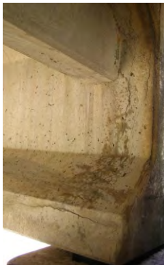
a) PC-I girder cracking
