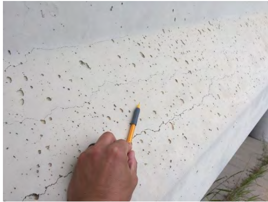
a) PC-I girder cracking
