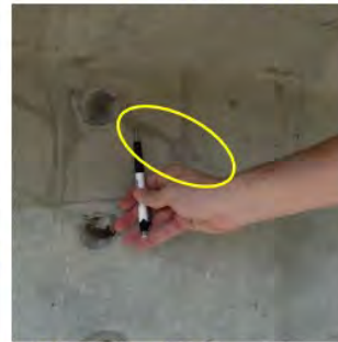
Close-up views of the diagonal crack
