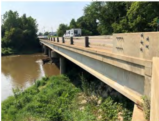
(b) Bottom flange of south fascia beam
