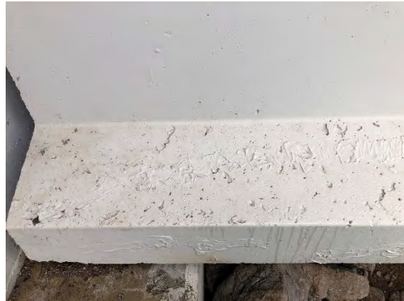
(b) Epoxy injected and repaired cracks
