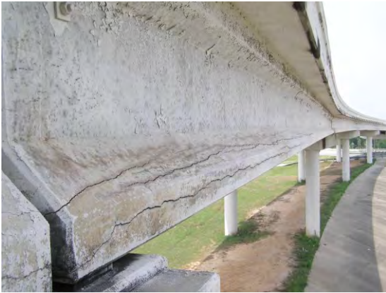
a) PC-I girder cracking
