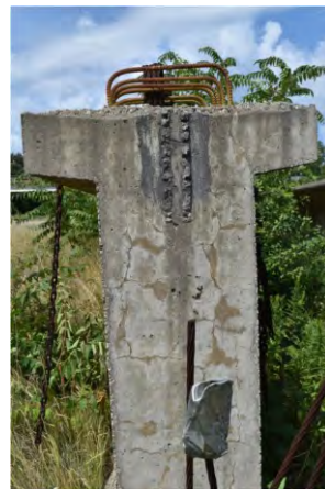
Map cracking on web
