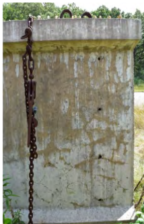
Map cracking on web
