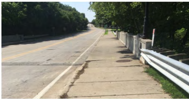
(a) General view of the bridge
