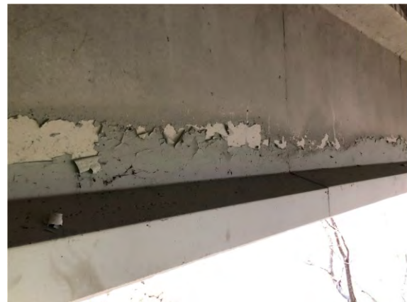
(d) Surface coating on the interior surface of the fascia
