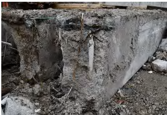
Figure D-3. Severely deteriorated beam ends (north end of the bridge)
