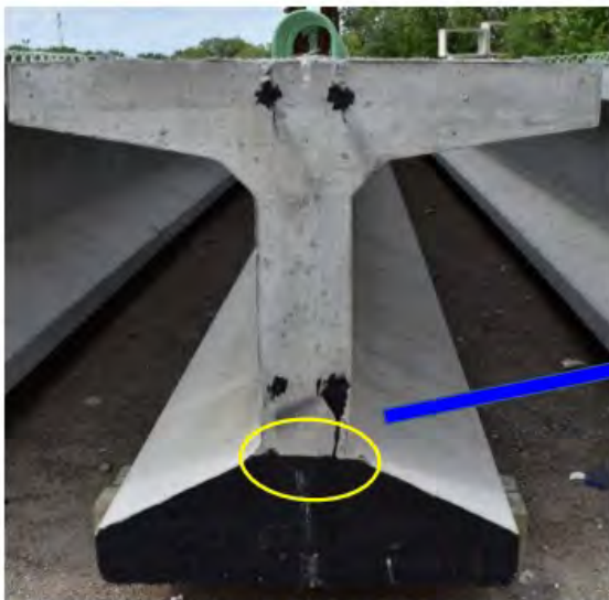
Cross-section of a bulb-tee girder
