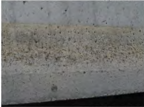
(b) Bottom flange map and longitudinal cracking
