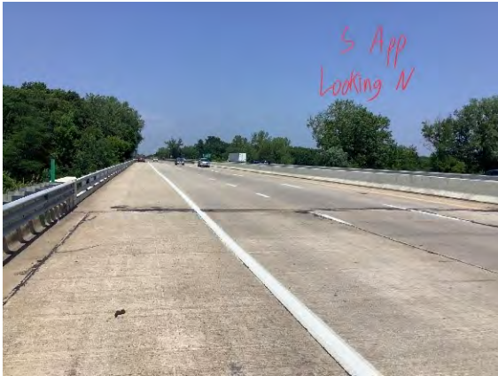
(a) General view of the bridge
