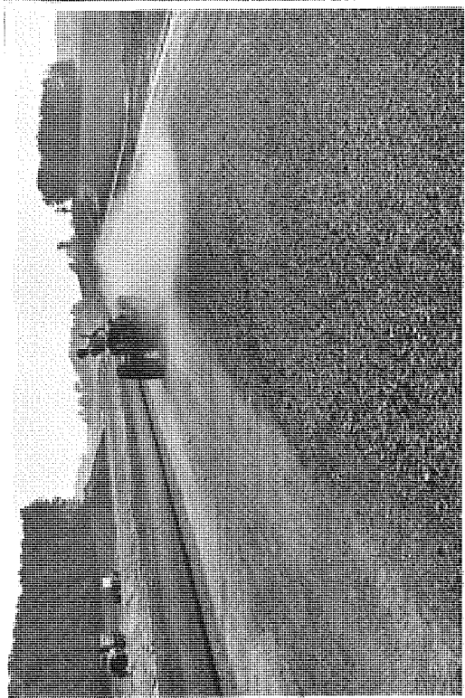
Figure 5 (left and right). Stabilized surface during and after brooming to remove stones and dirt. Note surface course in adjoining lane.
