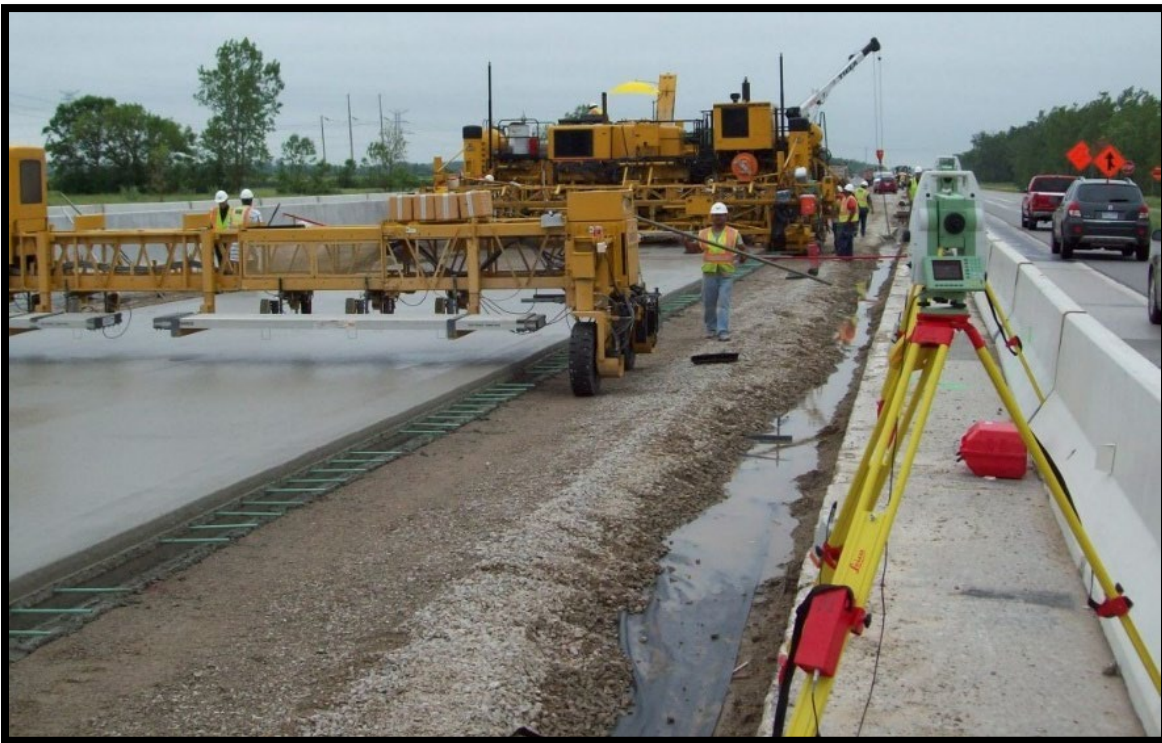
Figure 3. Example of AMG technology used for concrete paving.
