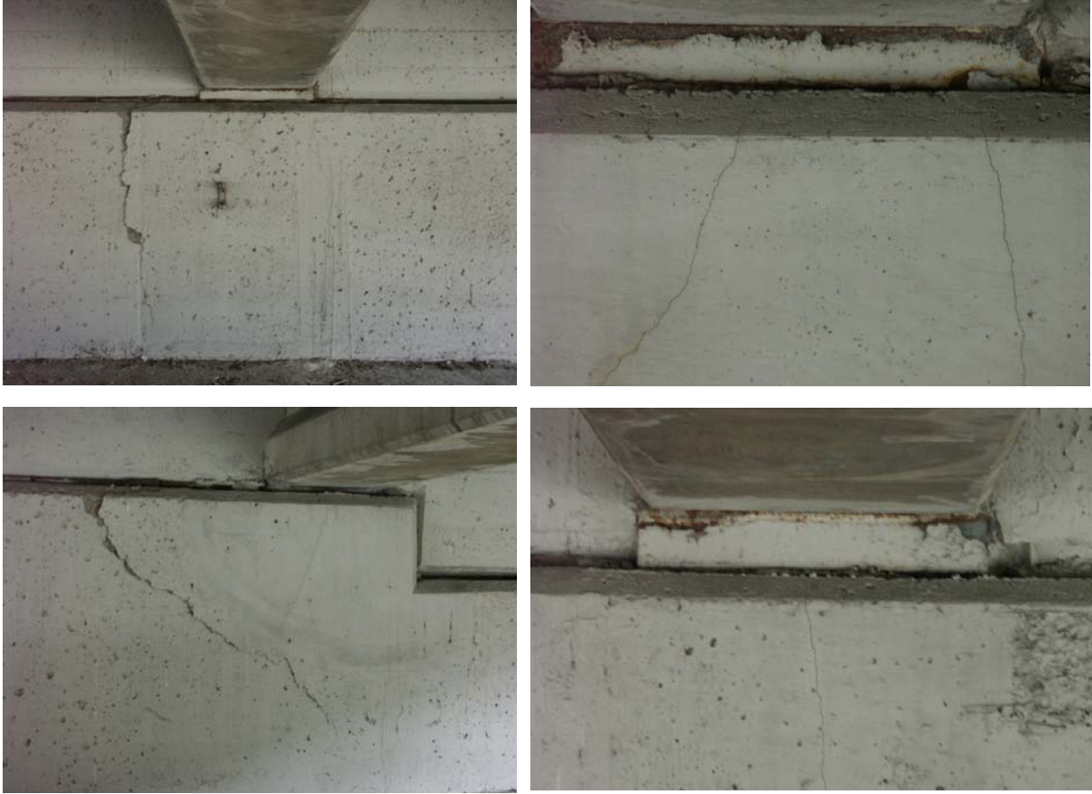
Photo C - 6. Abutment condition of I-75 north bound
