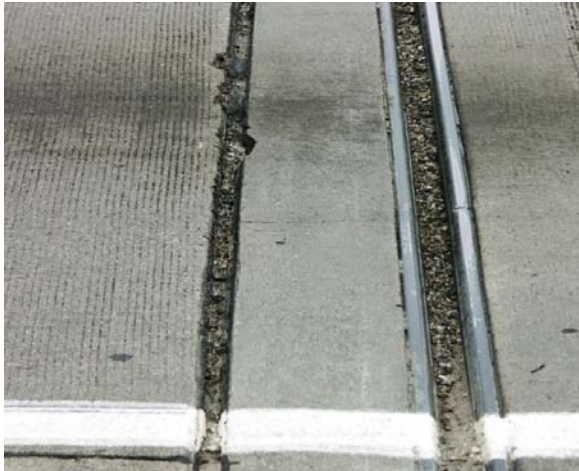
Photo C - 5. Sleeper slab condition (I-75 south bound)
