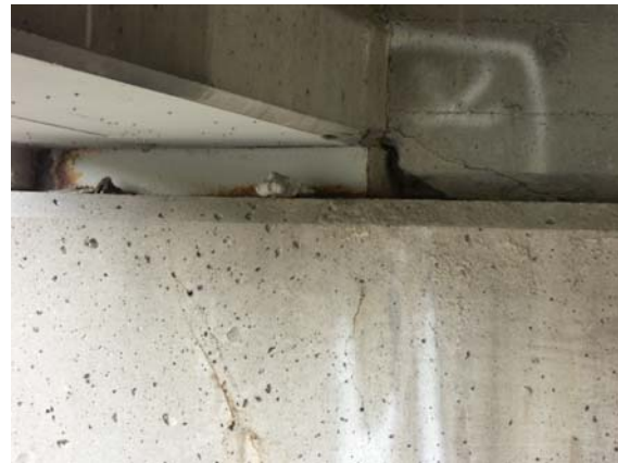
Photo C - 22. Transverse and diagonal cracks on I-69 EB bridge deck
