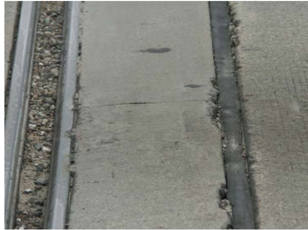
Photo C - 5. Sleeper slab condition (I-75 south bound)
