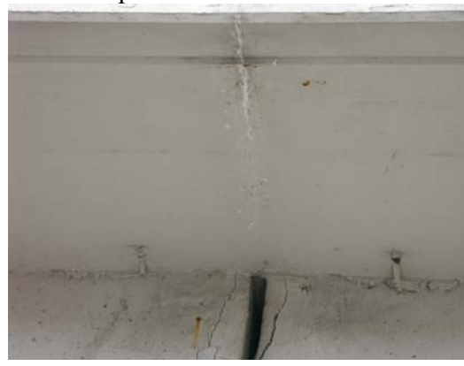
(a) Saw cut on the link slab above the pier centerline
