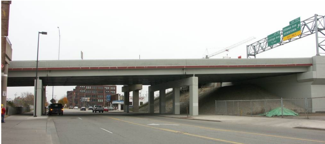
Photo C - 8. I-196 EB over Monroe avenue
