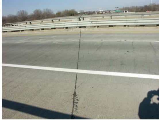
Photo C - 22. Transverse and diagonal cracks on I-69 EB bridge deck
