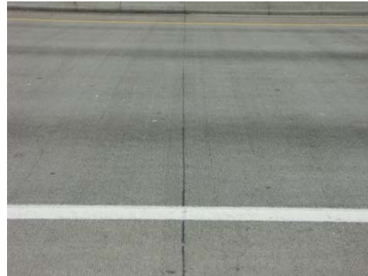
(a) Saw cut on the link slab above the pier centerline
