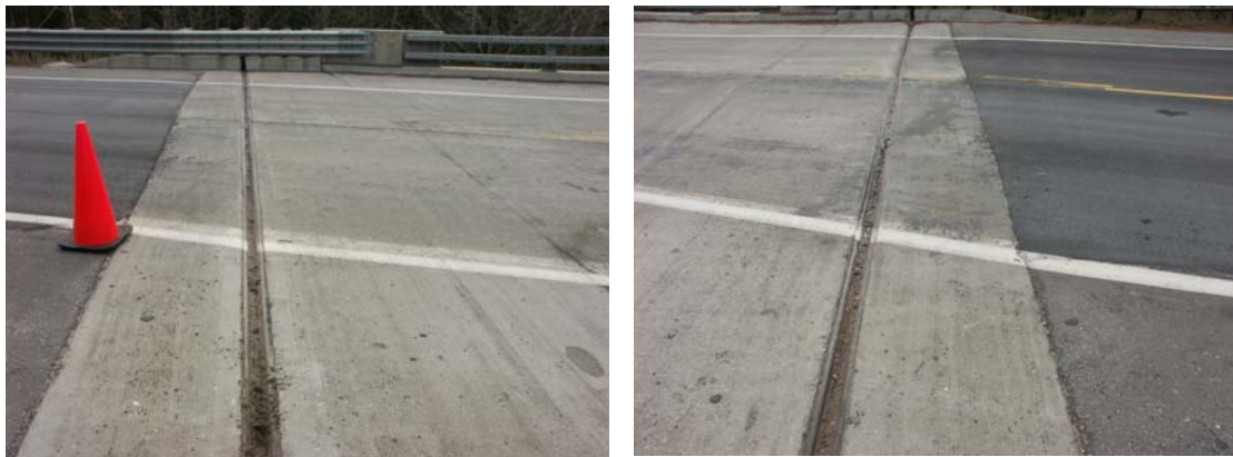
Photo C - 15. Expansion joints
