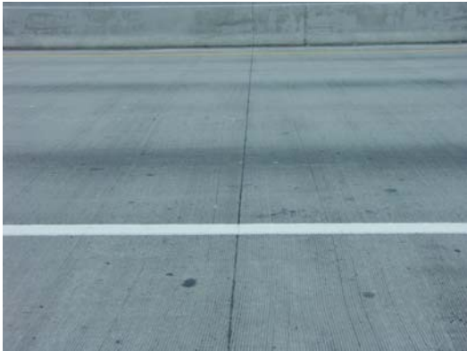
(a) Saw cut on the link slab above the pier centerline
