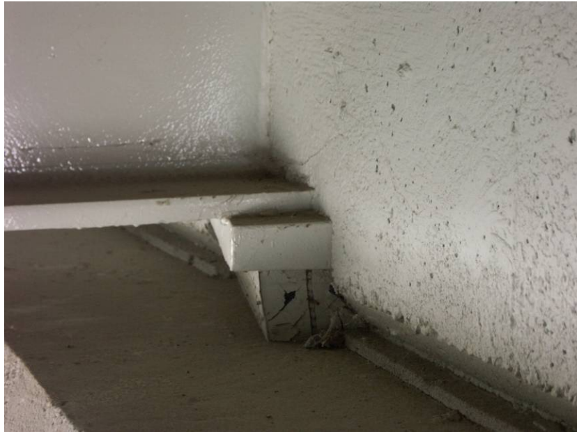
Photo C - 11. Deformed bearing
