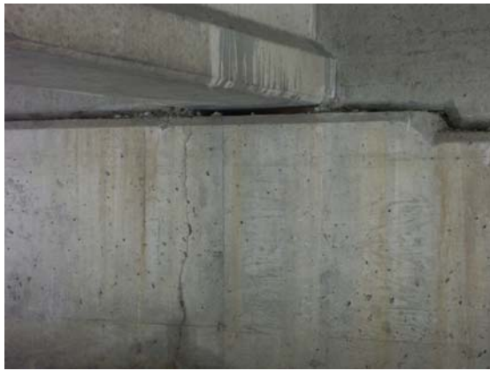
Photo C - 22. Transverse and diagonal cracks on I-69 EB bridge deck
