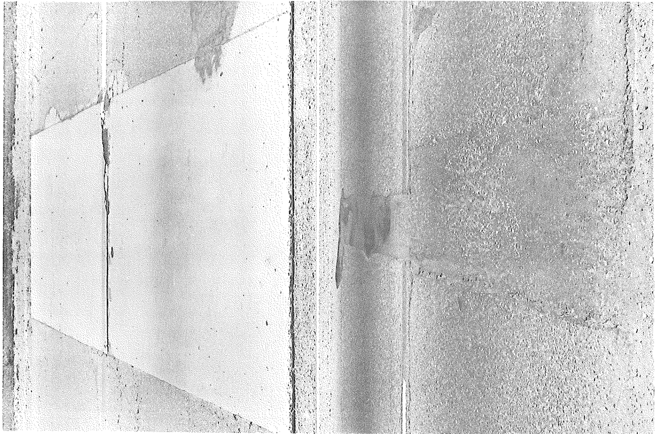
Figure 6 (left). Typical joint repairs in resurfaced pavement.
