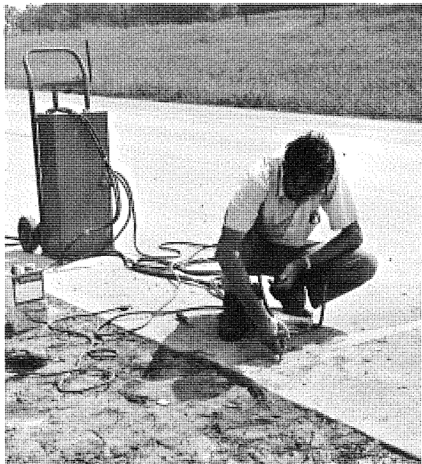
Figure 9. Injection of No. 1050 compressive epoxy.
