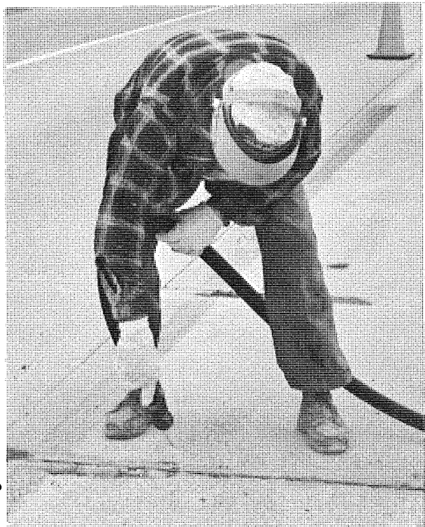
Figure 5. Close-up of cleaned joint groove.
