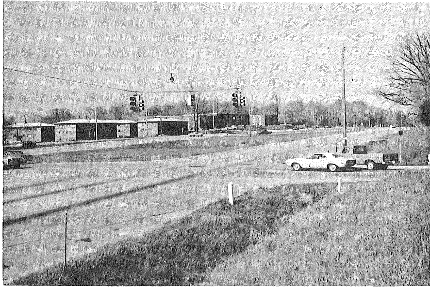
Typical rural high speed, divided roadway with narrow median. All red phase provides extra margin of safety between "near-side" and "far-side" signals.
