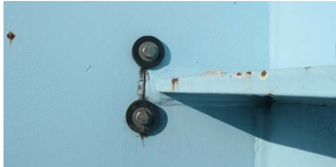
Figure 2-22. Drilled holes covered by bolts and nuts (Courtesy: Michigan DOT)
