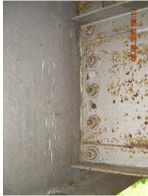
(a) Back side of the connection (view from abutment towards pier)
