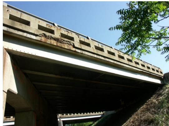
(b) Span 3 of I-94 EB over Puetz Road
