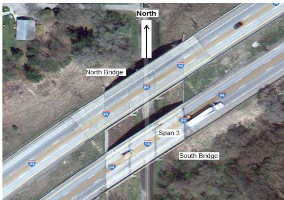
(a) Aerial view of I-94 over Puetz Road in Stevensville, Michigan
