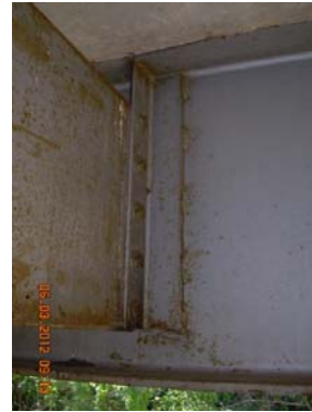
(b) Front side of the connection (view from pier towards abutment)
