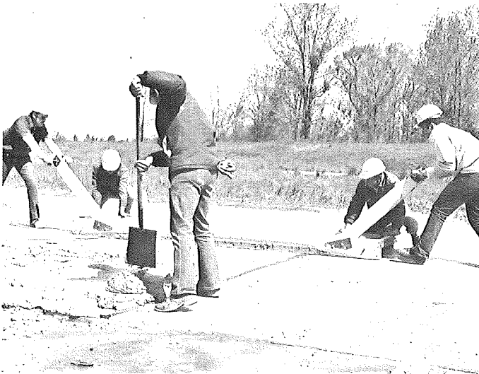
Striking of concrete with hand screed. Several passes are necessary to insure concrete is at the right elevation with respect to the existing slab.
