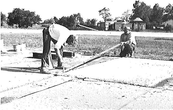
Removing wood strip used for forming joint groove. To prevent damage to the groove the strip should be removed 15 to 30 minutes after pour.
