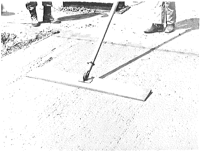
Finishing concrete surface with wood float.
