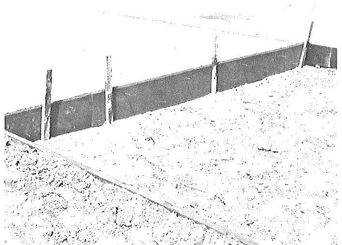
Polyethylene filler in place at repair using undoweled expansion joints. Note nails placed in filler for holding filler in place during cool weather the first year.
