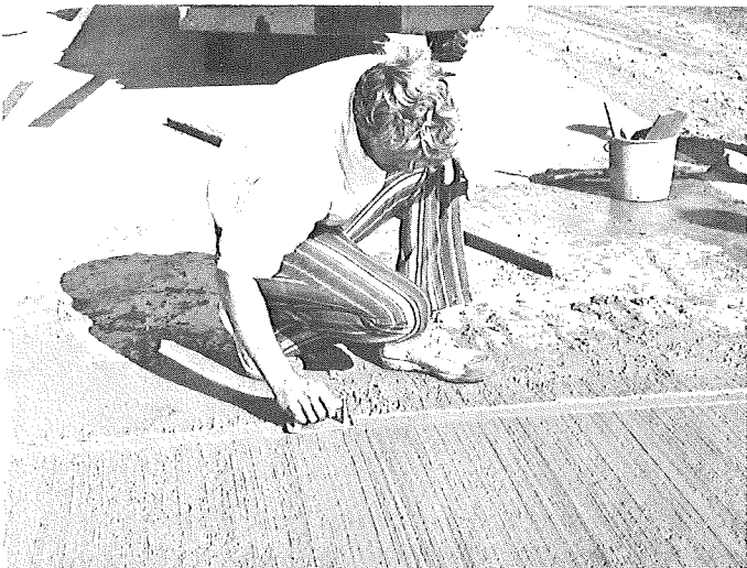
Edging repair slab along joint edge.
