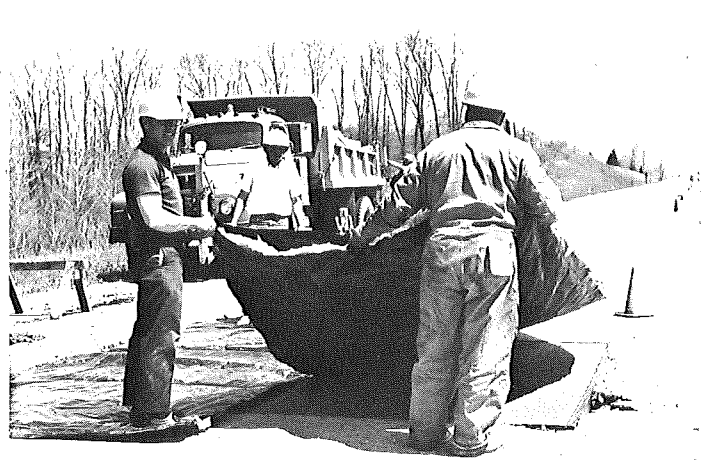
Curing blankets were used when the temperature was below 65 F.
