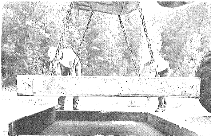
Placing precast slab with steel plate in its side for welding dowel to the slab.
