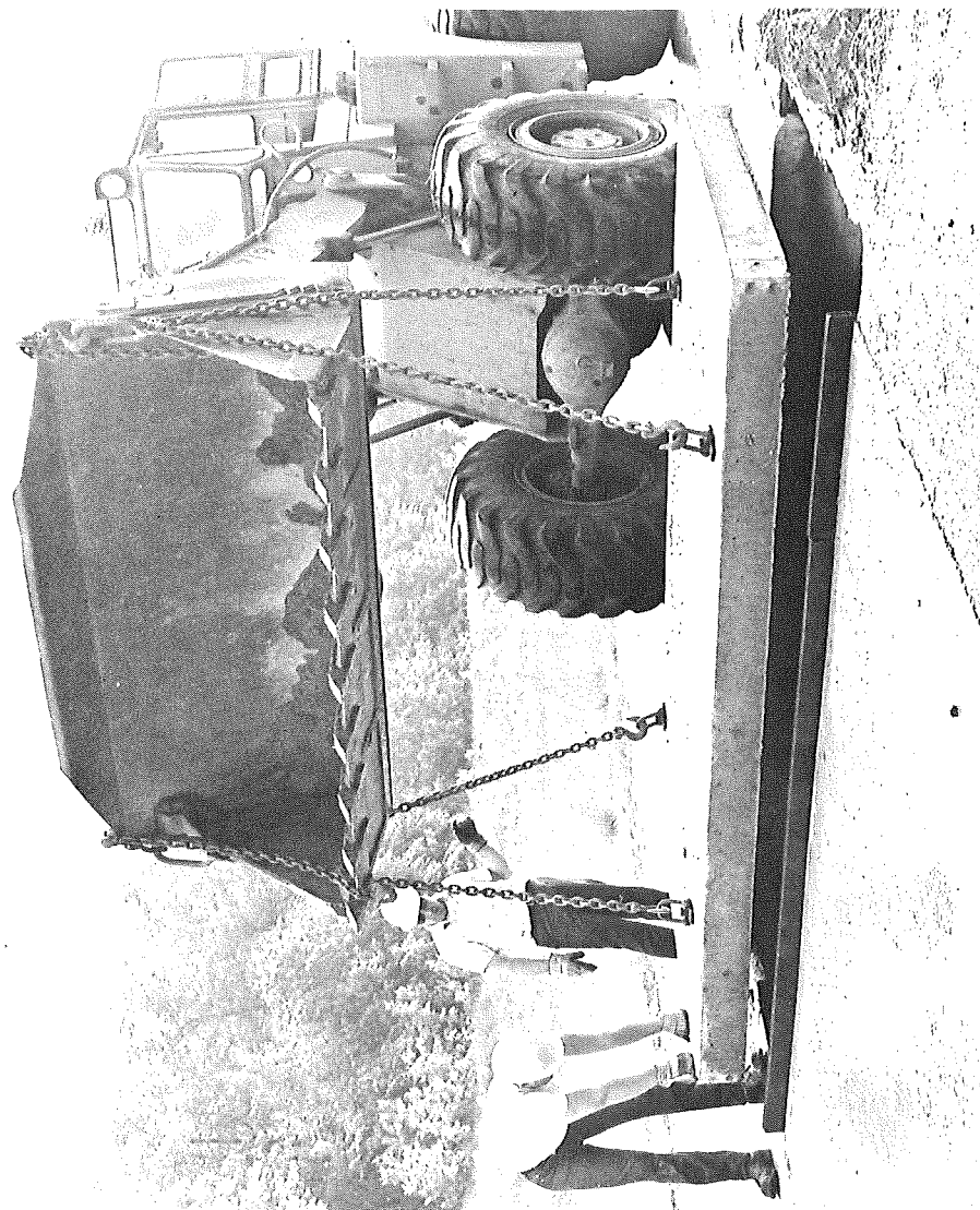
Figure 3B. One-inch, 'Type S' pickup insert with 1-in. coil and foam plug (upper left). One-inch, 4 lb swivel lifting plate being attached to insert cast into slab with 1 by 5-in. coil bolt (bottom left). Lift hook-up arrangement on front-end loader (above).
