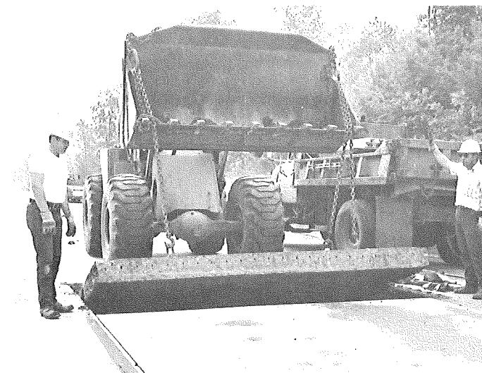
Removing second half of distressed concrete.
