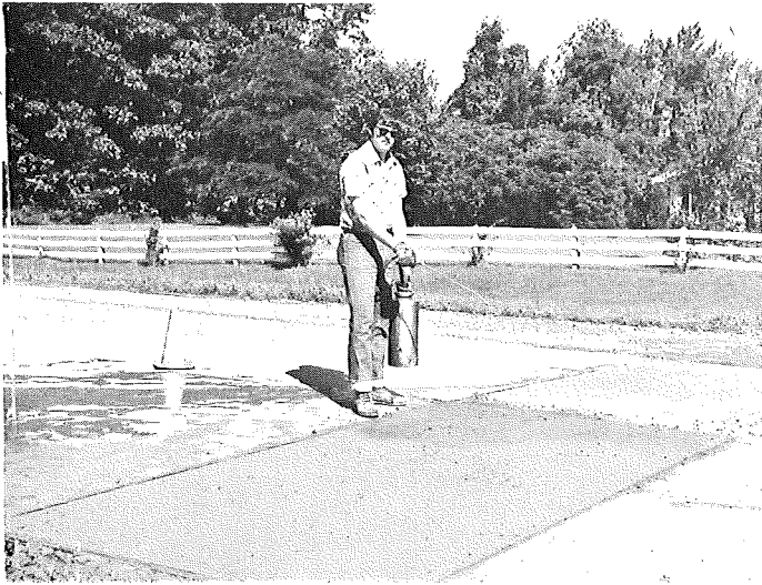
Applying curing compound with hand sprayer.
