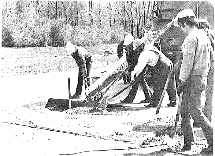
Pouring and vibrating concrete.
