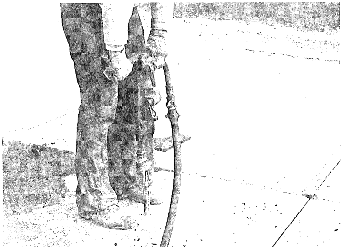
Drilling 2-in. diameter holes for lift pins. Normally four holes were used at each repair. Holes must be located in sound concrete areas.
