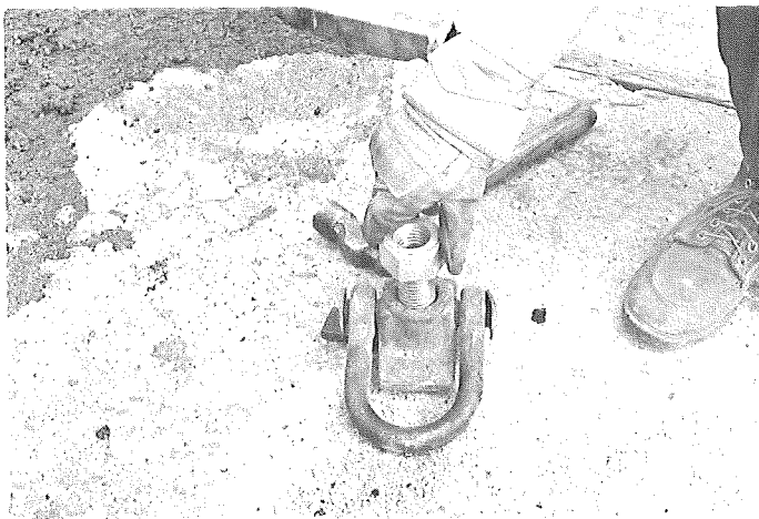
Installing lift pin. The pin itself is first placed in the hole, then the key is tapped in place, the swivel plate positioned over the pin, and the nut screwed on the bolt.
