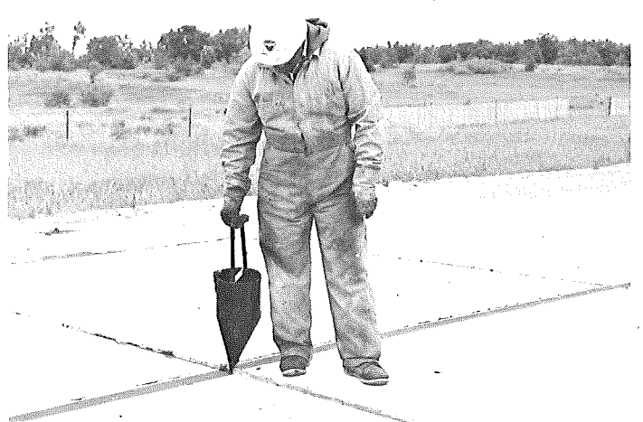
Sealing joint with hot-poured rubber-asphalt sealant.
