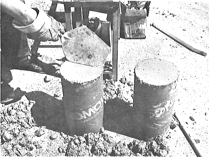
Preparing concrete cylinder for compressive strength tests.
