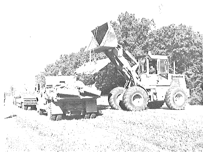
Loading deteriorated concrete onto dump truck.
