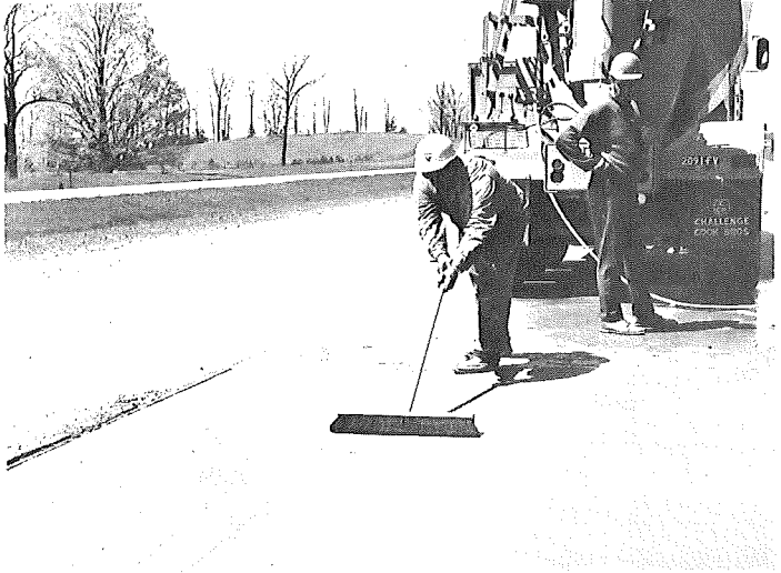
Applying broom finish to slab.
