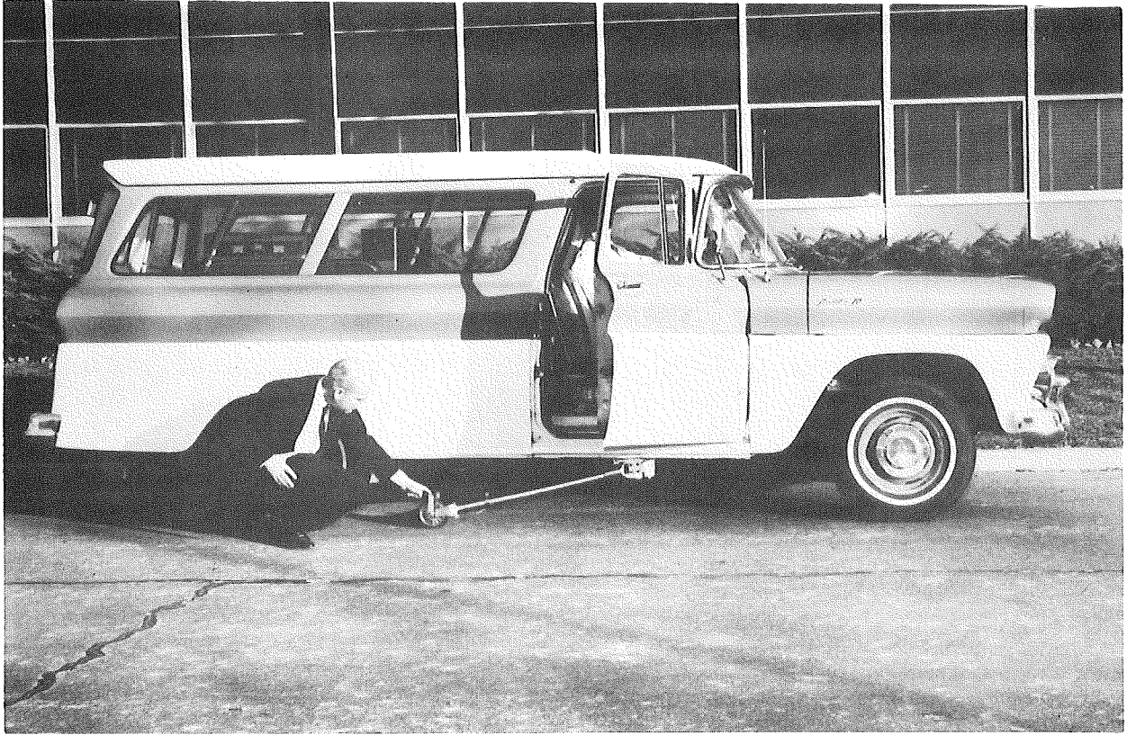
Figure 1. The General Motors rapid travel profilometer.
