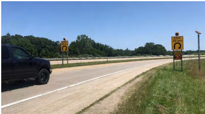
c. DSFS 450 ft Upstream of Curve (Under Existing Curve Warning Sign)
