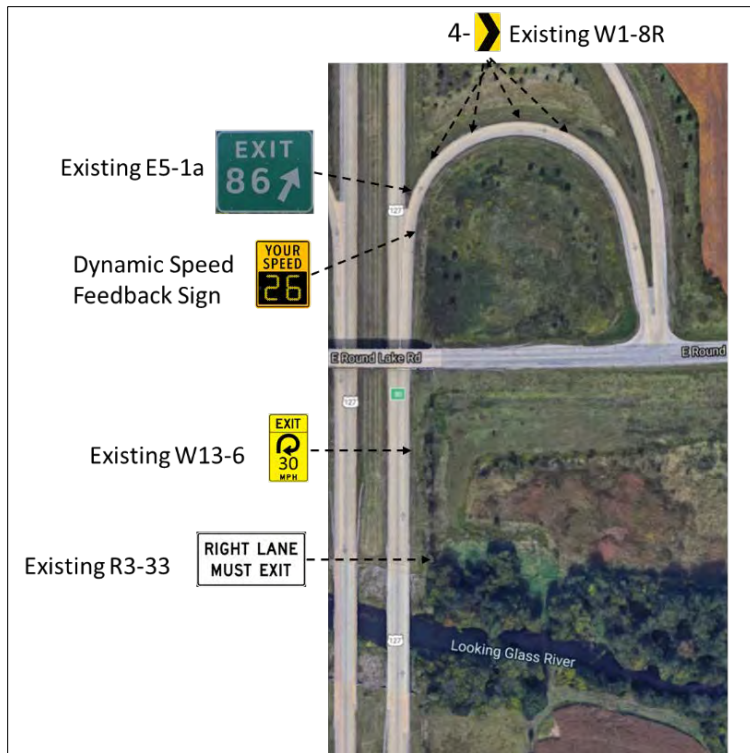
Figure 16. NB US-127 exit ramp to Round Lake Rd (Site 3)
