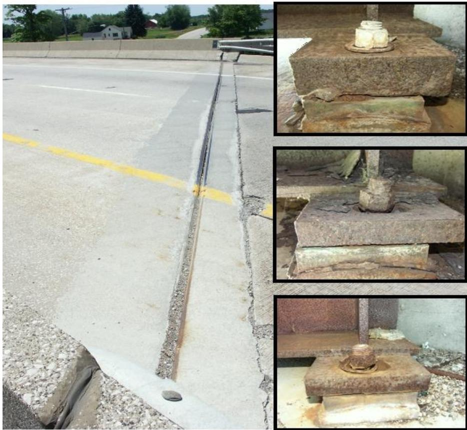
**Figure 3-11. Expansion bearing and joint condition at south abutment**
