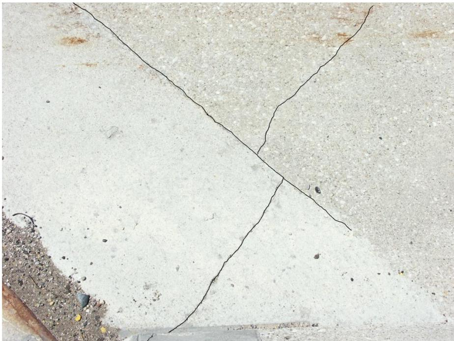
(c) Deck cracking close to the obtuse corner of the deck over south abutment
