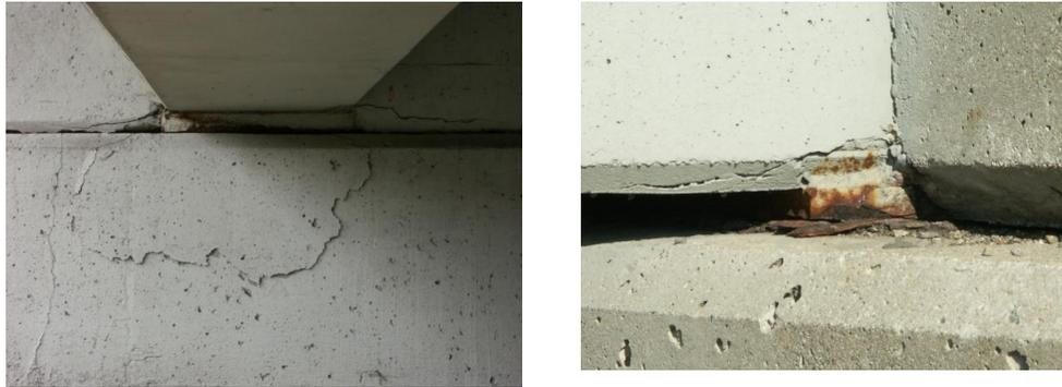
**Figure 5-16. Abutment and girder end distress**
