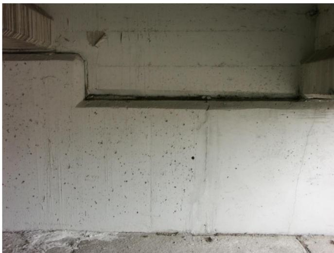
**Figure 2-53. Backwall and abutment configuration of a bridge with different girder depths**
