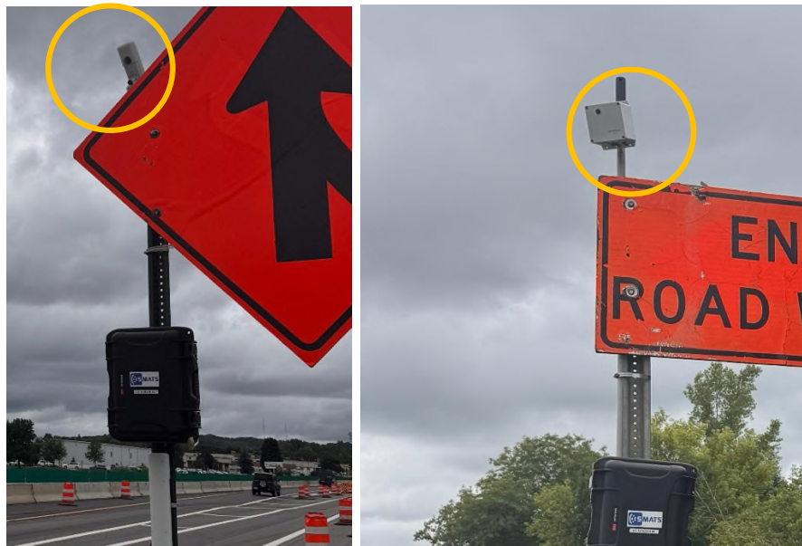
Figure 6-3 Field sensor installation for video camera data collection
