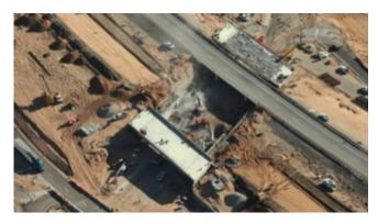
One method of accelerated bridge construction involves building a new bridge alongside the bridge to be replaced. The new bridge is moved quickly into place after the old one has been demolished.
