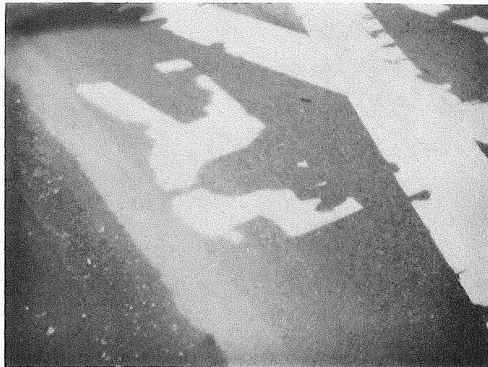
Considerable chipping has taken place with a good pavement surface. This could be the result of poor adhesion or snow plowing.
