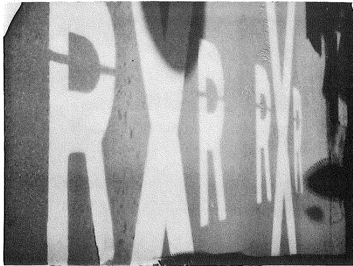
Close up of marking in photo above Note the excellent condition of the pavement surface
