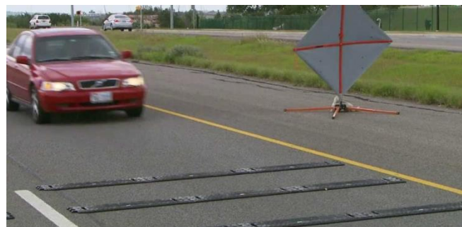
Figure 21. Installed Portable Temporary Rumble Strips (Photo Credit: Antigo Times)
