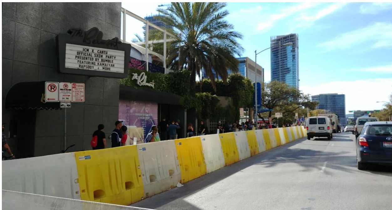
Figure 37. Pedestrian Bypass Channelization Using Water-Filled Barriers (Photo Credit: City of Austin)
