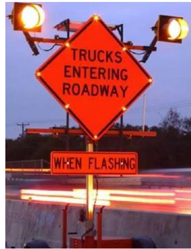
Figure 13. Truck Entry Warning System
