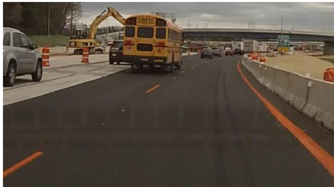
Figure 2. Orange Temporary Marking on Asphalt Surface
