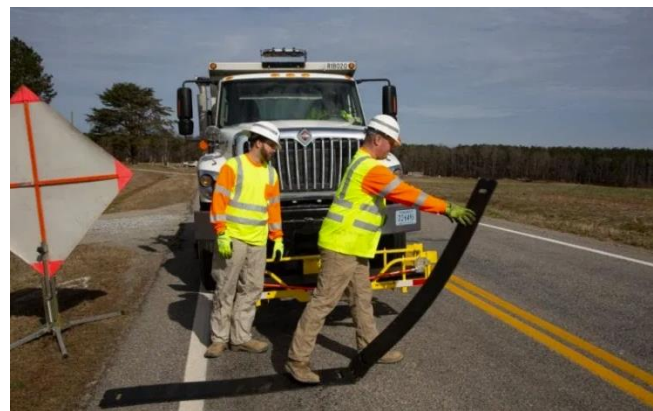
Figure 22. Installation of Portable Temporary Rumble Strips (Photo Credit: Augusta Free Press)
