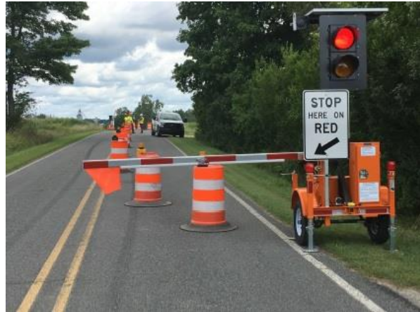
Figure 11. Closed Lane AFAD Application in Michigan
