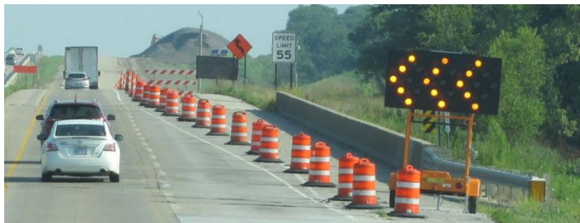
Figure 6. Traditional Freeway Lane Closure Using an Arrow Board
