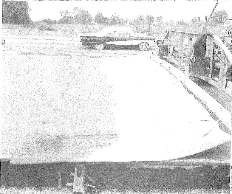
Figure 16. Applying burlap drag finish to concrete surface.
