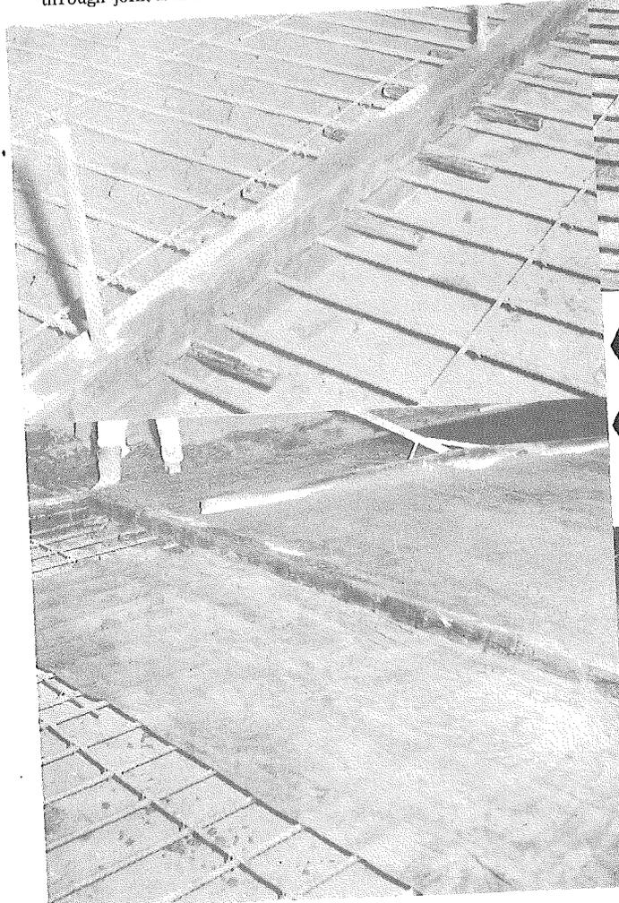
◀ Figure 22. Continuous bar mat reinforcement in place through joint header.
