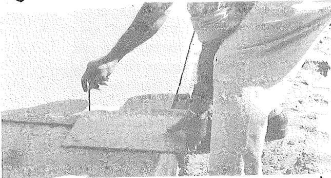
Figure 30. Finishing concrete surface after setting plugs.
