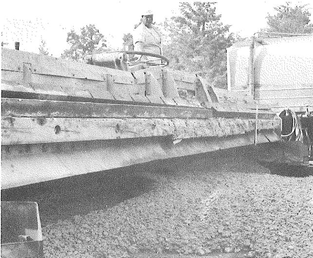
Figure 8. Spreading and striking off concrete with Blaw-Knox spreader.
