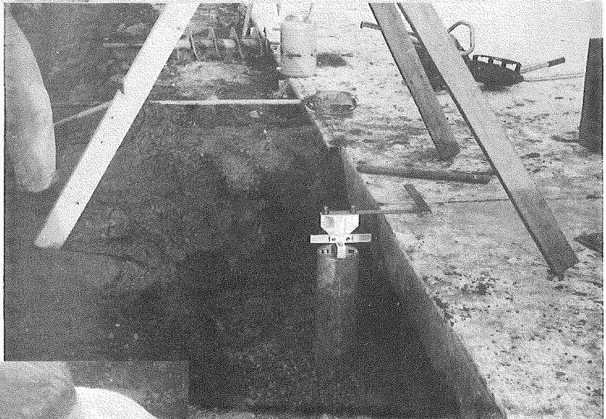
▶ Figure 42. Setting monument for absolute slab displacement.
