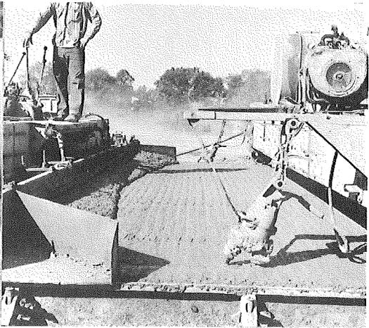
Figure 13. Initial finishing of concrete surface with Jaeger-Lakewood finishing machine.
