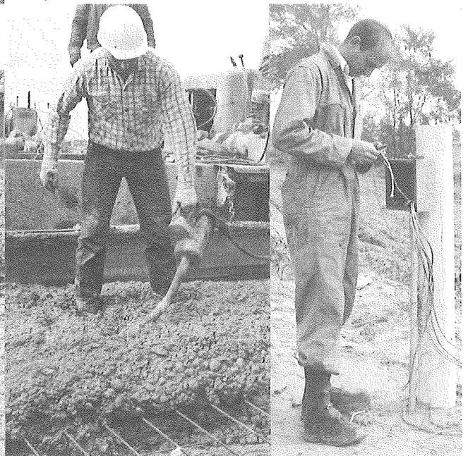
Placing Plugs for Absolute Slab Movement. One gage plug was placed in the concrete after the final hand finishing operation, 4 in. from the ends of the continuously reinforced sections and 12 in. from the pavement edge in the passing lane. Similarly, a gage plug was installed 4 in. from the beginning joint of the ten consecutive contraction joints in the standard section.
