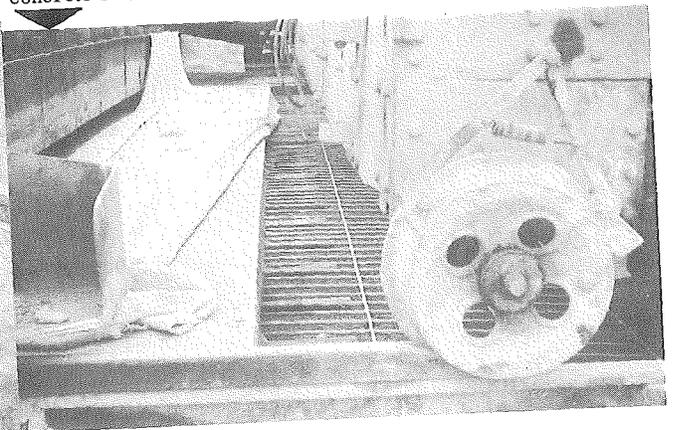
The portion of the reinforcement extending through the joint was supported on boards which kept the steel level and made it easier to align the dowel bars. The concrete was hand vibrated throughout the width of the joint and about 5 ft back along the side forms. Burlap was placed over the extended reinforcement to catch excess concrete spilling over the header during finishing operations. Construction is shown in Figs. 19 through 24.
