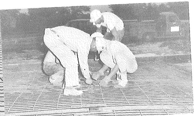
▲ Figure 20. Wiring dowel bars to wire mesh reinforcement.
