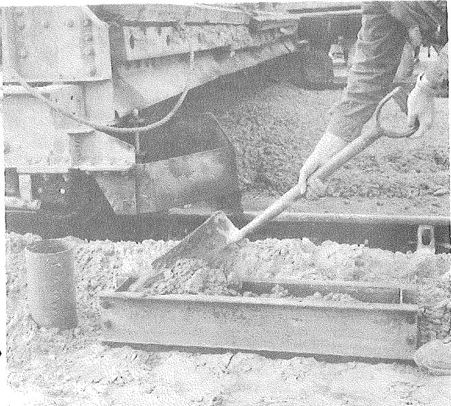
Figure 28. Taking beam samples for modulus of rupture tests.
