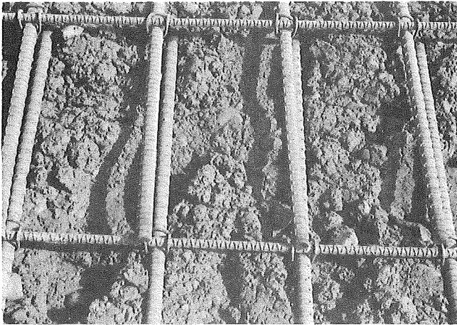
Figure 6. Lap in continuous bar mat reinforcement.
