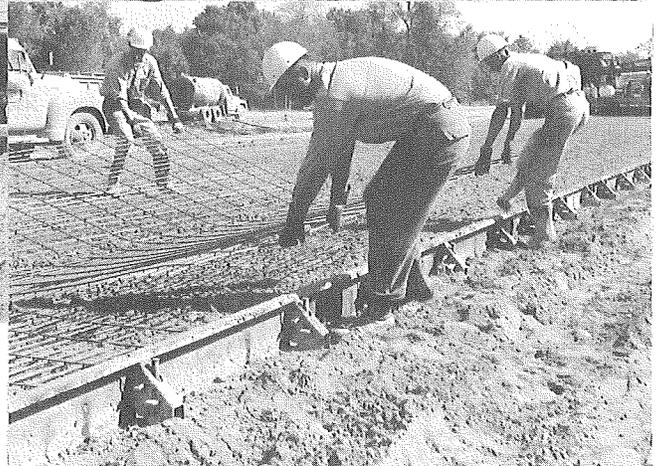
Figure 10. Placing bar mat reinforcement in continuous section.
