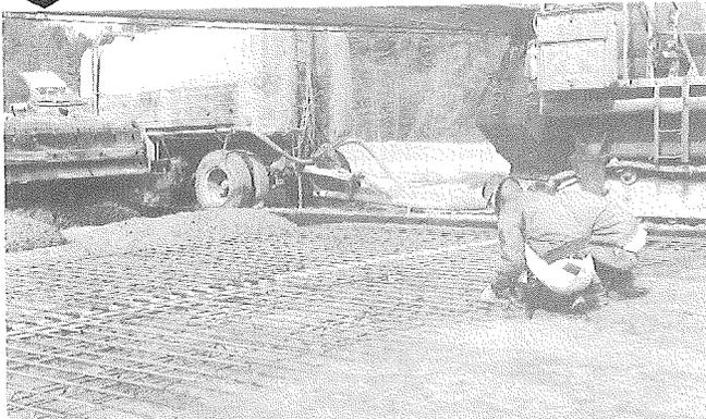
Figure 33. Placing plastic tube containing thermocouples in subbase.
