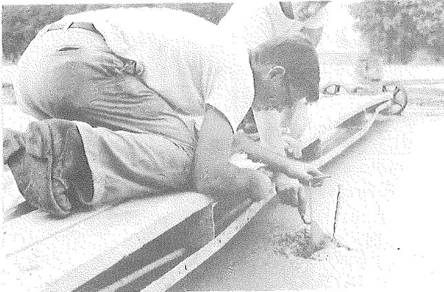
Figure 27. Taking slab temperature and steel depth measurements.
