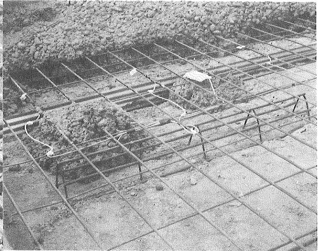
Figure 35. Instrumented standard mesh reinforcement with corrugated crack former.
