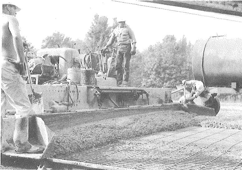
Figure 12. Spreading concrete with Jaeger-Lakewood finishing machine in continuous wire mesh section.
