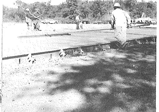
Figure 15. Final hand finishing of concrete surface.
