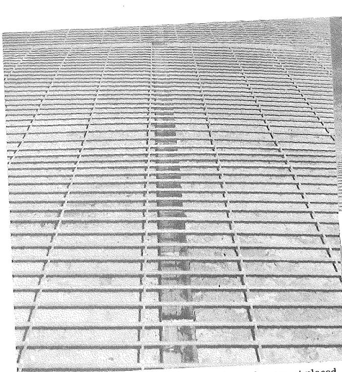
▲ Figure 19. Continuous wire mesh reinforcement placed over lower set of 4 by 4's
