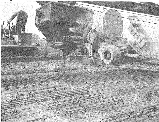
Figure 38. Pushing concrete into instrumented standard mesh reinforcement.
