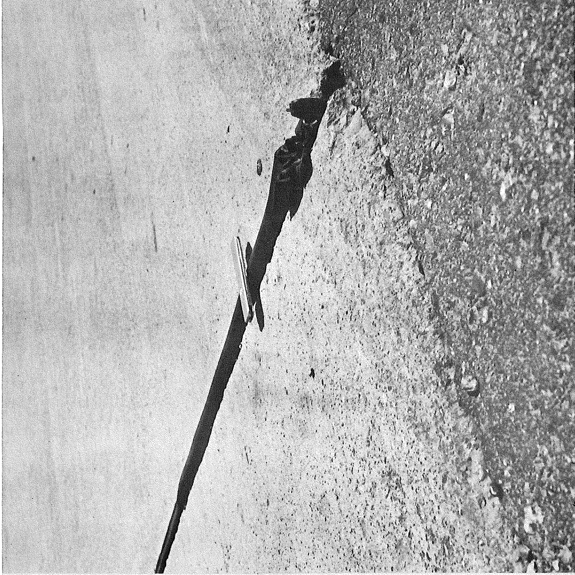
Figure 1. Contraction seal with 2-in. long break.
