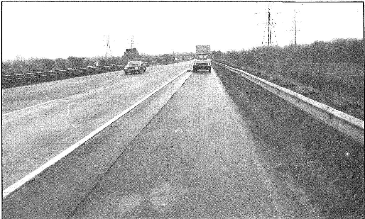
Figure 5. Two-foot bituminous strip in shoulder next to the concrete pavement (project 4).
