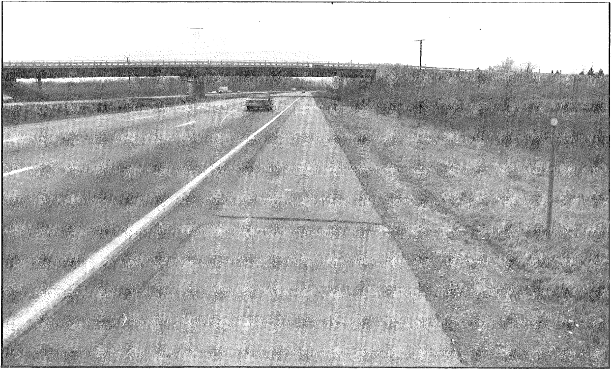
Figure 6. Two-foot bituminous strip next to pavement edge and two-foot bituminous strip leading to edge of shoulder for retrofit drainage system (Northbound roadway of project 10).
