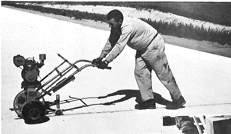
Figure 4. Crimping the Unitube.
