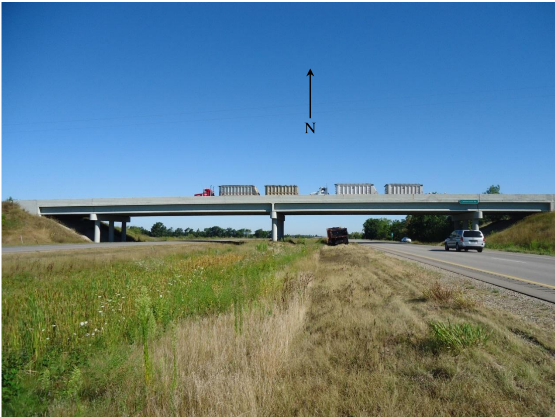
Figure 6.15. Following Test Trucks In Center Of Bridge.
