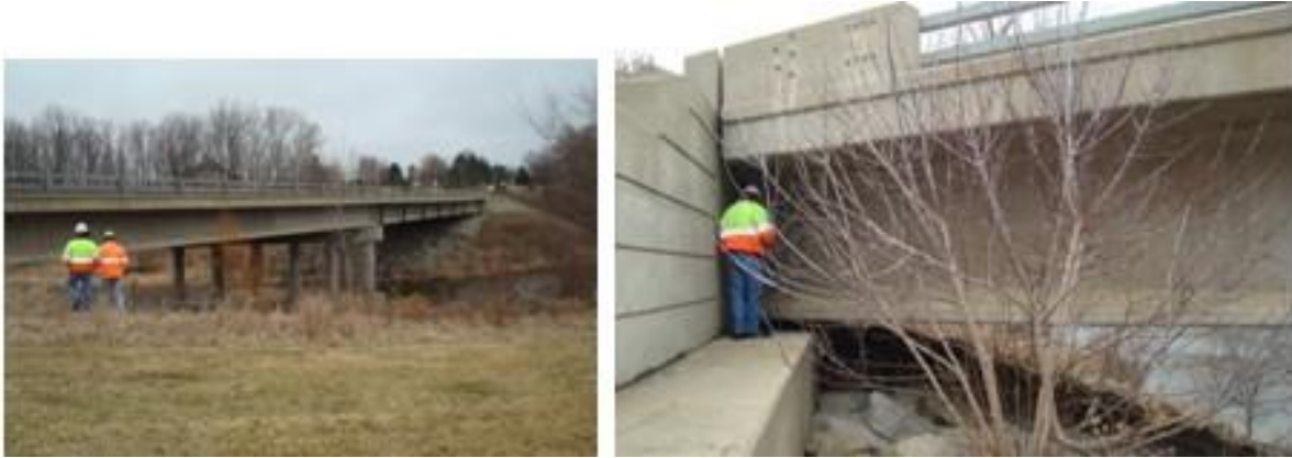
Figure A63. Bridge 16 (#9728).
