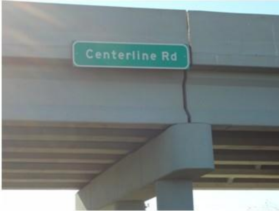
Figure A75. Bridge 19 (#12773).
