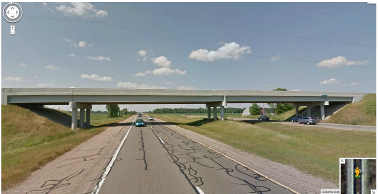
Figure 6.3. Bridge 2, Taft Road Over US-127.
