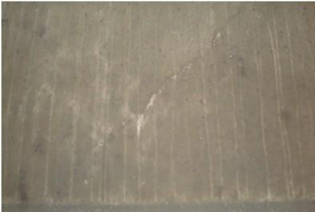
Figure A11. Crack diagram for south span girder, north end, 4 th beam from east side, west face (#7933).
