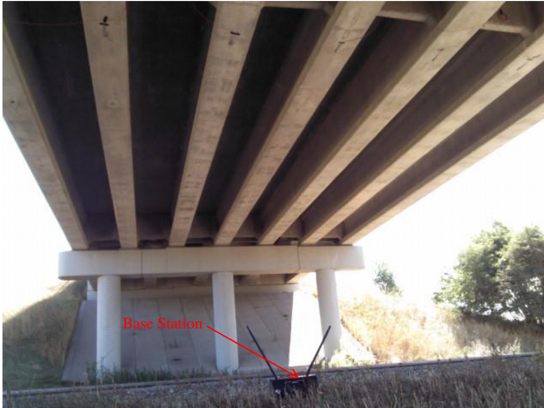
Figure 6.10. View Of Bridge With Base Station And Attached Gages.
