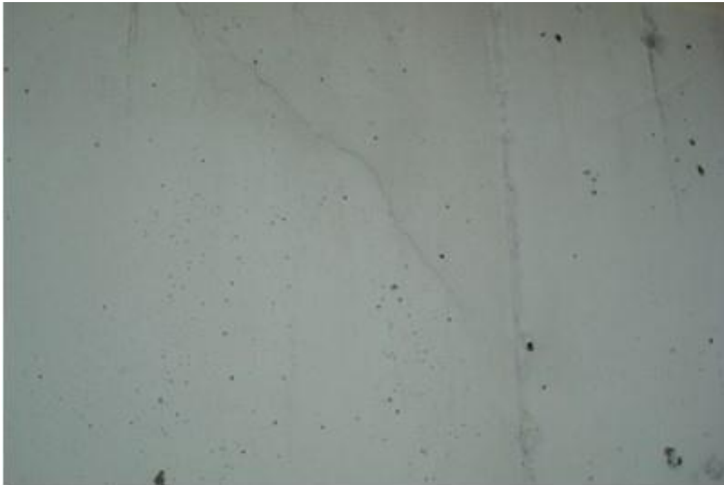
Figure A17. Cracks on south span girder, exterior beam, west side, interior face (#7933).
