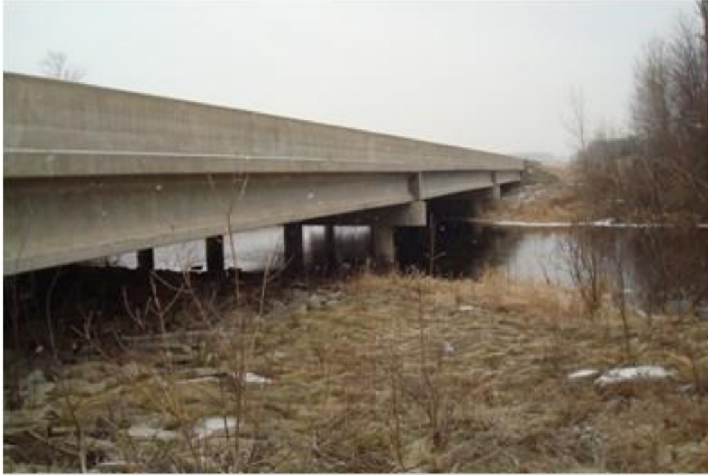
Figure A72. Bridge 18 (#12693).
