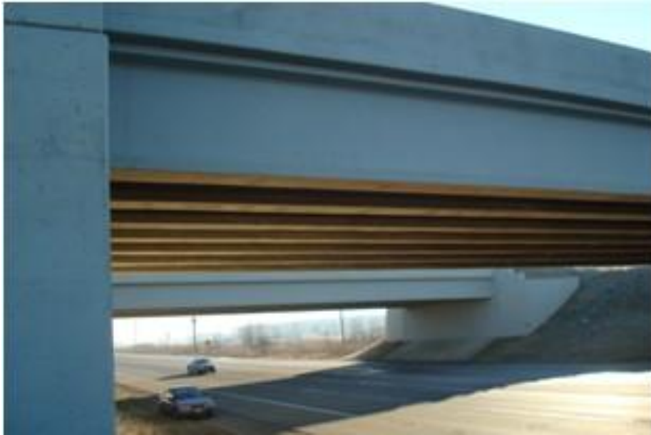
Figure A38. Bridge #5 (#1829).
