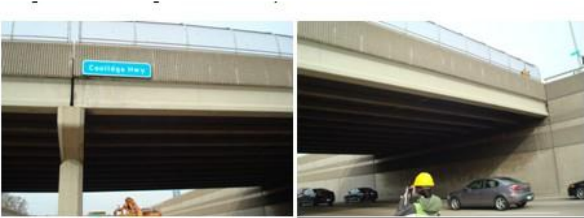
Figure A1. Bridge 1 (#7933).
