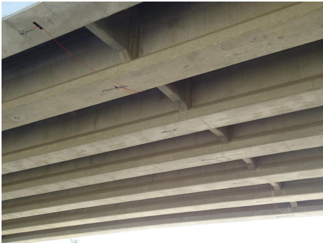
Figure 6.9. View Of Bridge With Gages Installed.
