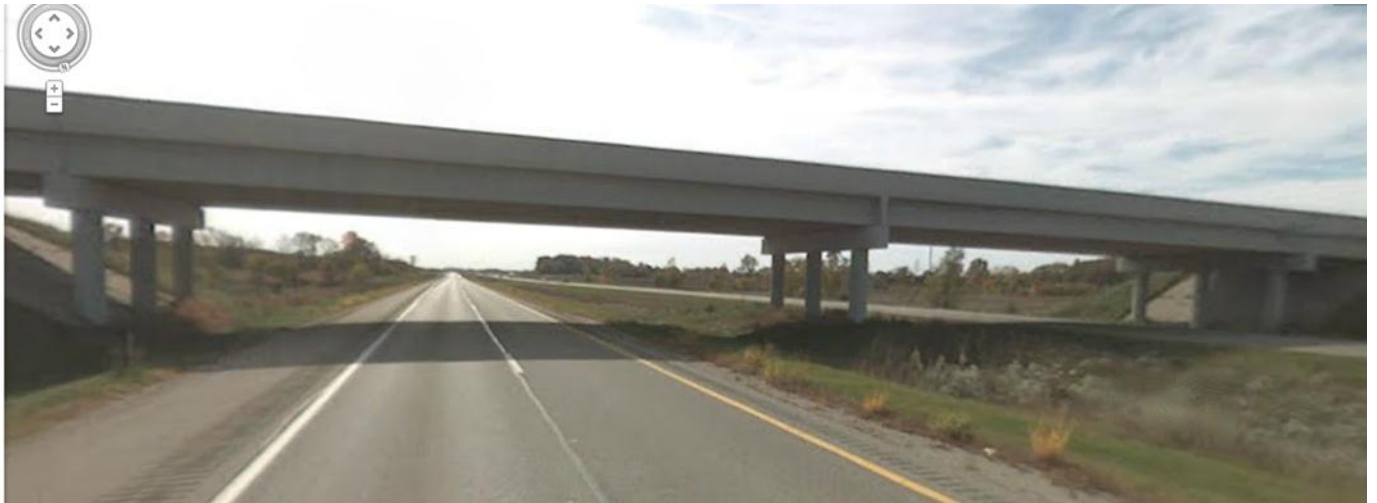
Figure 6.2. Bridge 1, Centerline Road Over US-127.
