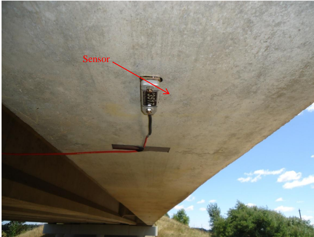
Figure 6.8. Gage Installed On Girder.
