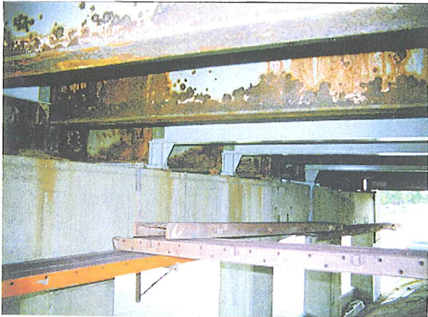
Figure 5 - Pier 1 of S05 of 63022 prior to coating
