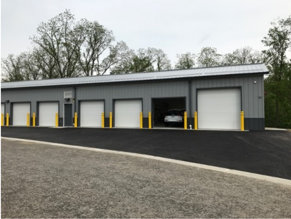
Figure 29: The exterior of the Mcity garage upon completion.
