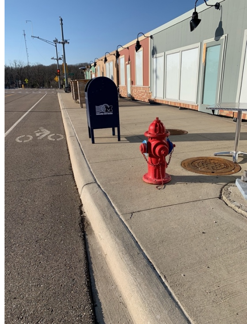
Figure 21: Examples of items regularly found along the roadside (mailbox, fire hydrant) and squared curbing.
