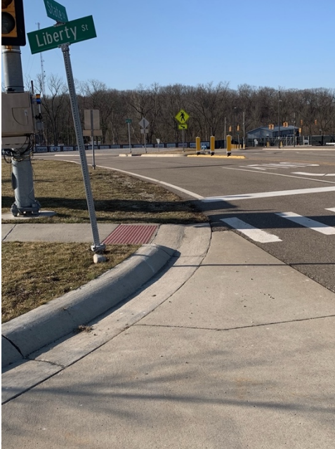
Figure 12: Examples of pavement transitions (asphalt to gravel and concrete to asphalt) and a low sloping curb.
