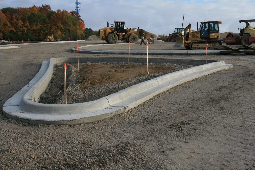
Figure 2: Roundabout under construction, Fall 2014.
