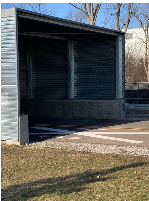
Figure 15: Entrance to tunnel producing sharp transitions in light level and attenuating wireless signals.
