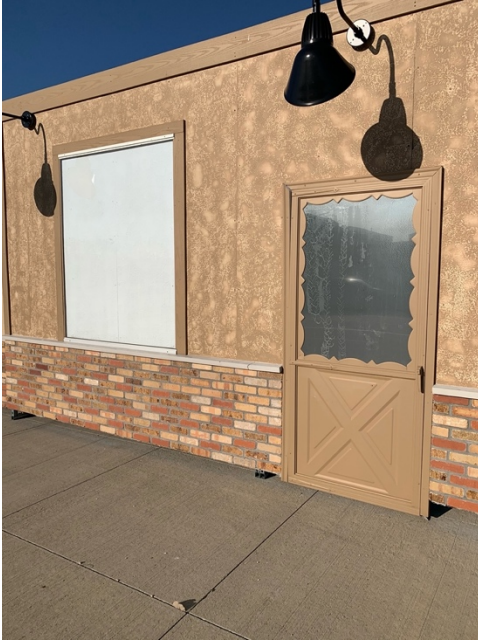
Figure 20: Examples of real construction materials used in building facades (brick, glass, aluminum, cement board).
