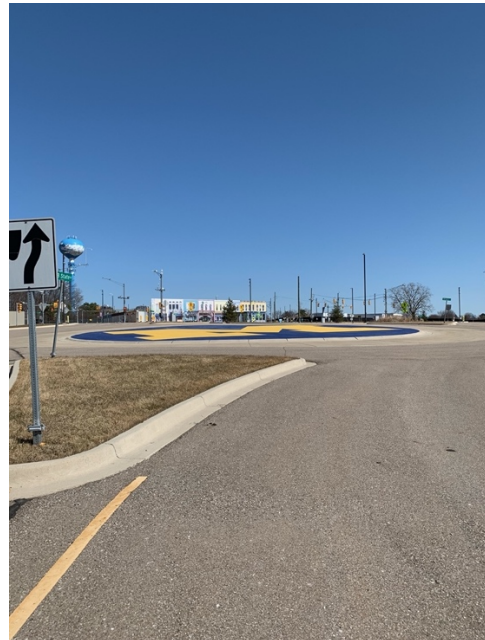
Figure 18: Roundabout on a compound slope with unevenly distributed entrance and exit points.
