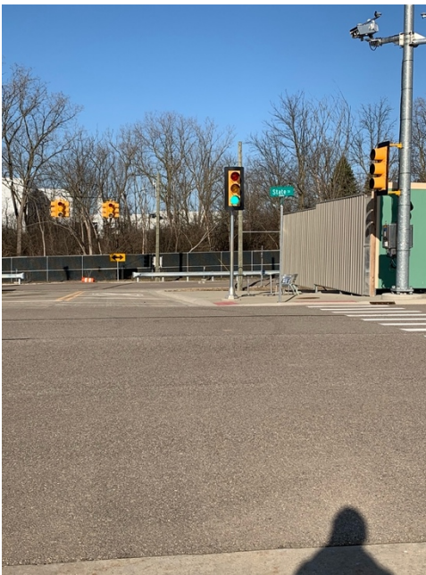
Figure 9: Examples of post- and pedestal-mounted traffic signal heads as well as suspended from wooden poles.
