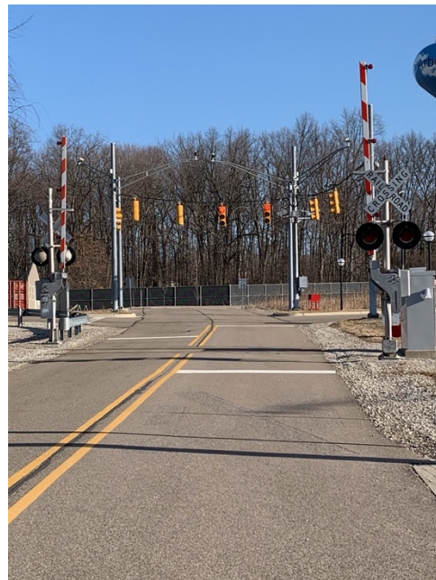
Figure 11: Gated railroad grade crossing and traffic signal heads suspended from metal poles.
