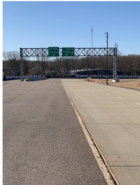
Figure 23: Concrete and asphalt pavement and highway signage on a truss.
