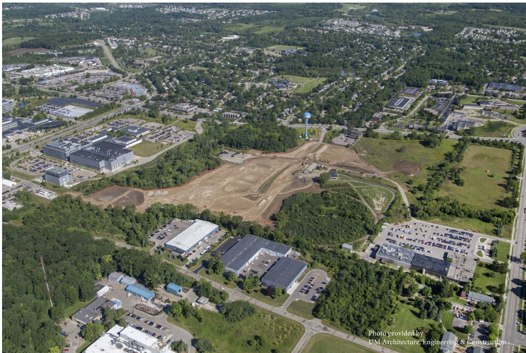
Figure 1: Aerial photo of Mcity under construction, Summer 2014.
