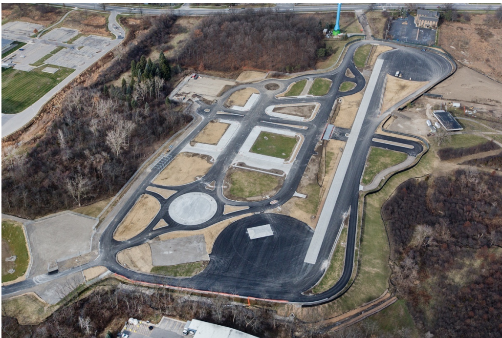
Figure 3: Aerial photo of Mcity under construction, Spring 2015.
