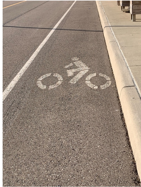
Figure 10: Bicycle lane surface markings and square concrete curb.
