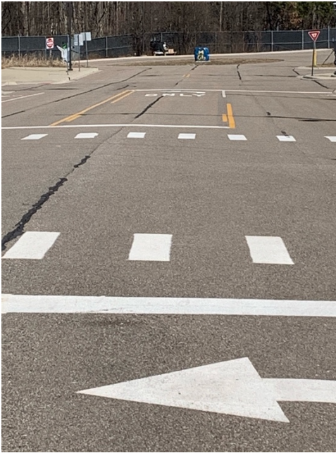
Figure 8: Various lane marking materials (latex-based paint and thermal plastic) and a traffic circle.
