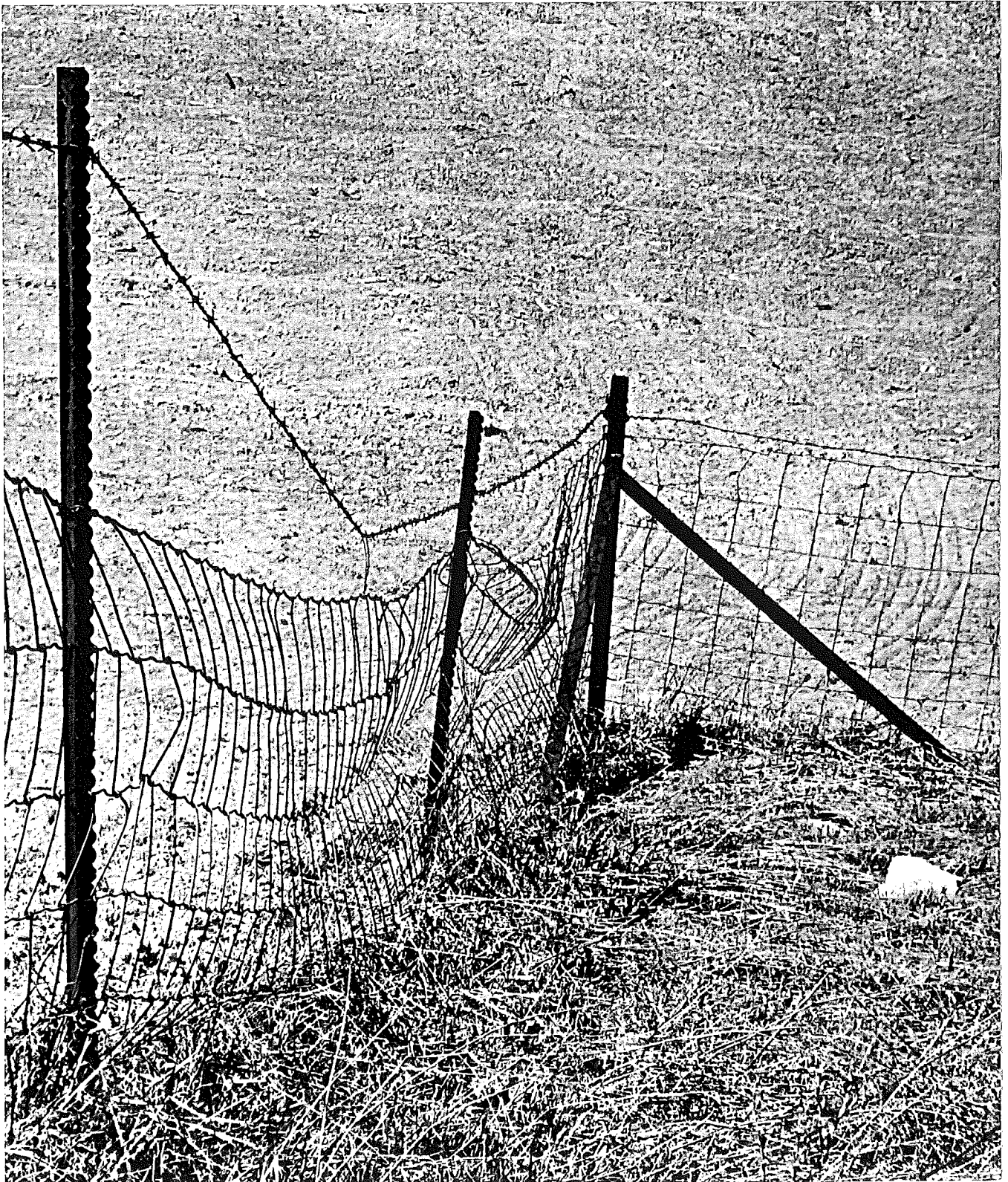
Enlargement made from preceding photograph to illustrate tie clips missing from posts.
