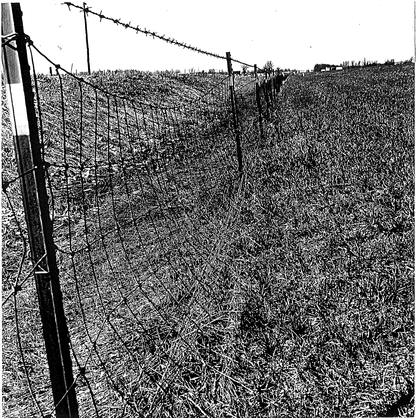
View of fence facing north from post shown in preceding photograph. Note bulging of fence wire at bottom, suggesting movement of heavy snow masses; also that post lugs in general have served their purpose well.
