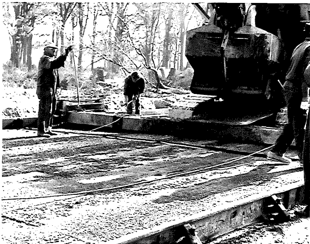
Figure 4. At a typical joint the base plate is placed on the subbase (left), and the two joint dowel assemblies are positioned over the plane-of-weakness strip (center and right).
