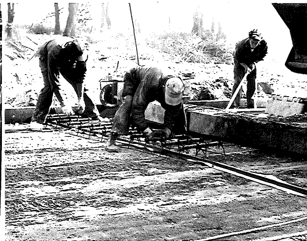
Figure 4. At a typical joint the base plate is placed on the subbase (left), and the two joint dowel assemblies are positioned over the plane-of-weakness strip (center and right).
