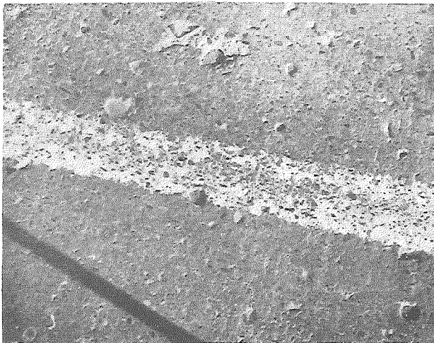
◀ STRIPE 32, NORTH WHEEL TRACK . NORTH LANE, 50% REMAINING. PAINT F
