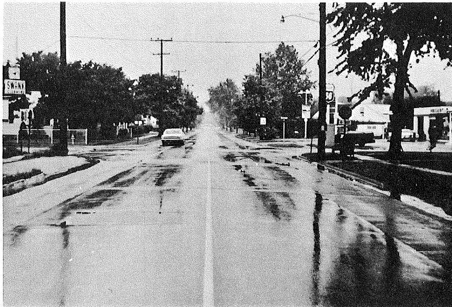
NORTHBOUND THIRTEENTH STREET
