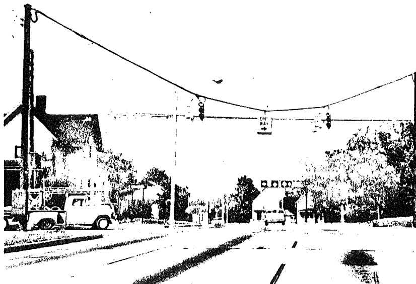
Figure 4-2. Traffic control signal installation with illuminated case sign.
