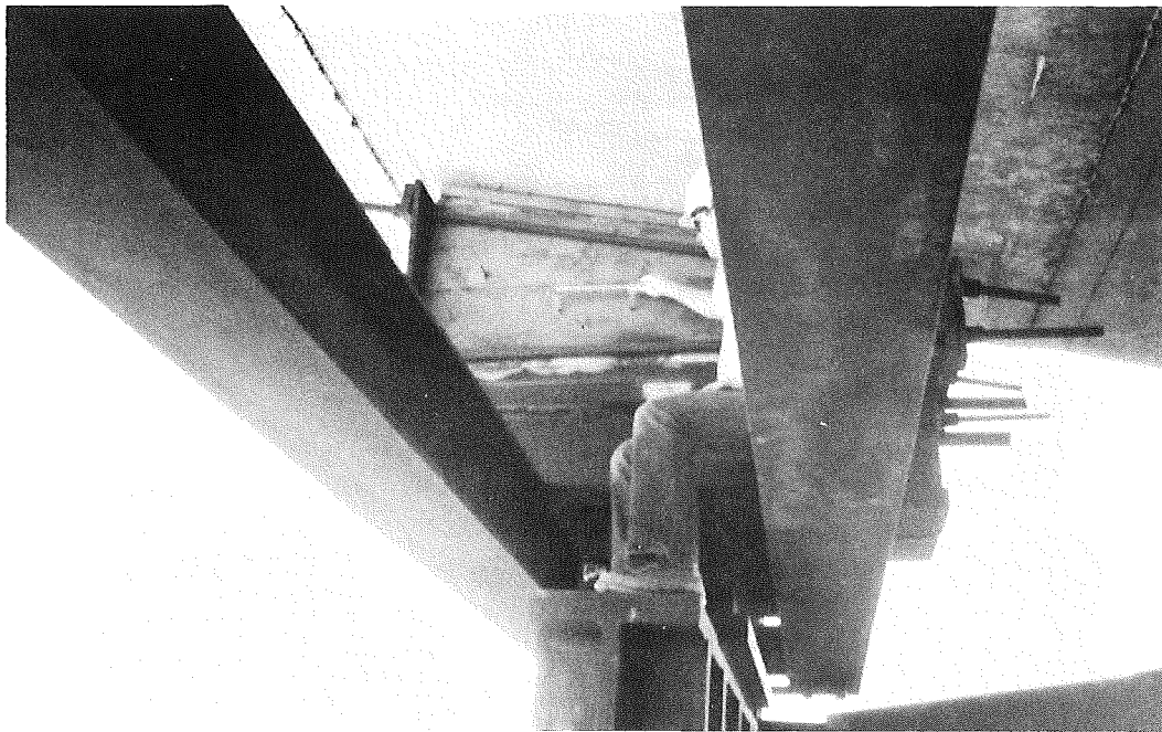
Figure 29. Calipers are used to monitor bearing block cracks.
