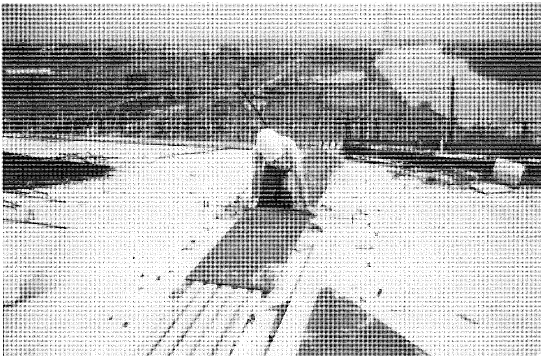
Figure B-22. Measuring expansion joint with trammel points.
