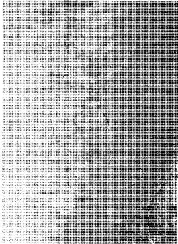
Figure B-12. Cracking in the original footing; north wall (upper left), west wall (lower left), and east wall (above).
