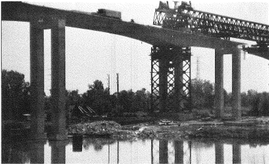
Figure 34. Zilwaukee bridge after completion of the realignment procedure.
