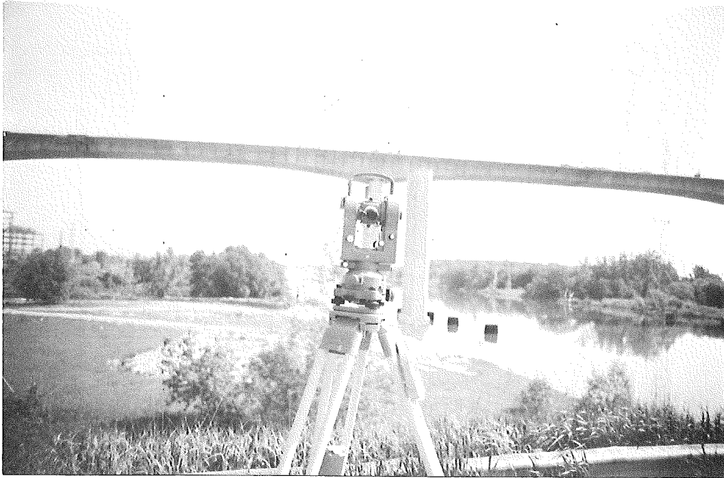
Figure B-23. A theodolite was used to monitor superstructure movement between piers.
