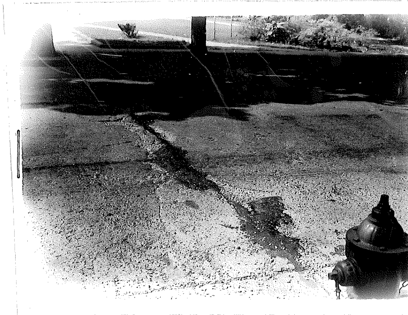
Figure 18. 73-11, C1 (1928) M 60, Three Rivers at Garden and Michigan Streets. Slight blowup at expansion joint. Note crushing and slight heaving of concrete. Similar conditions are no doubt responsible for heaving of bituminous capped projects.
