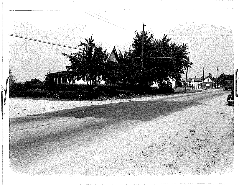
Figure 13. Project 11-3, C3 Benton Harbor East. Several old blowup areas were repaired by simply covering area with a huge patch of oil aggregate mixture without attempting to remove heaved concrete.
