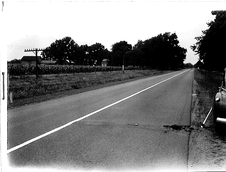
Figure 10. Project 78-14, Cl. White Pigeon Nest. Typical heave on this project. Area 24 inches wide 1 1/2 inches high, one side only.
