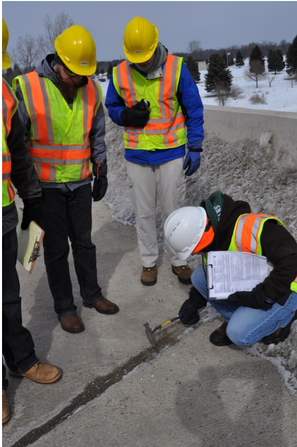
Figure 3-5: MTRI staff observe an MDOT inspector examining joint condition.
