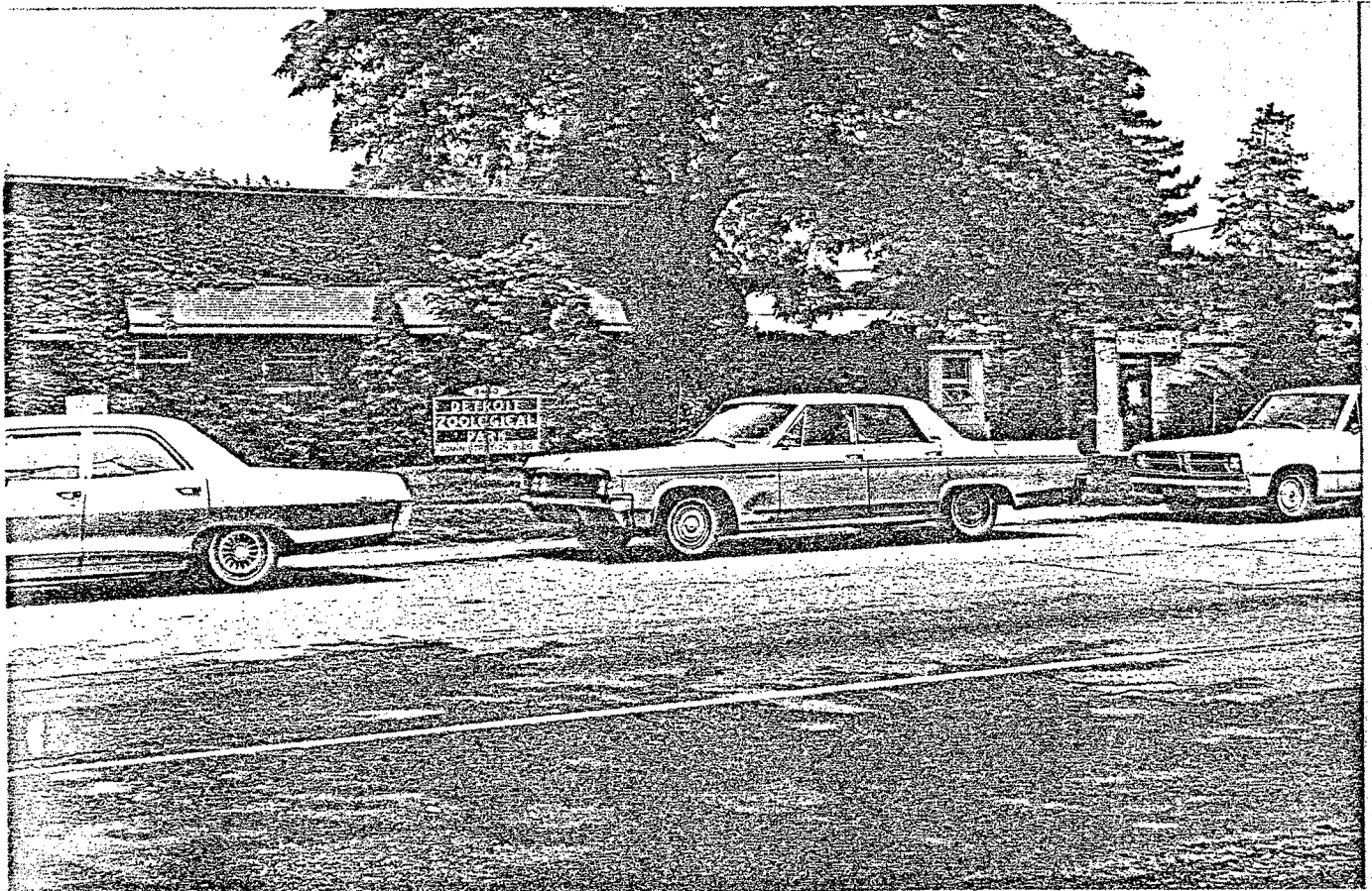
Figure 11. Microphone located 50 ft S of SW corner of Zoo Administration Building, observer looking NE. Sta. 312.
