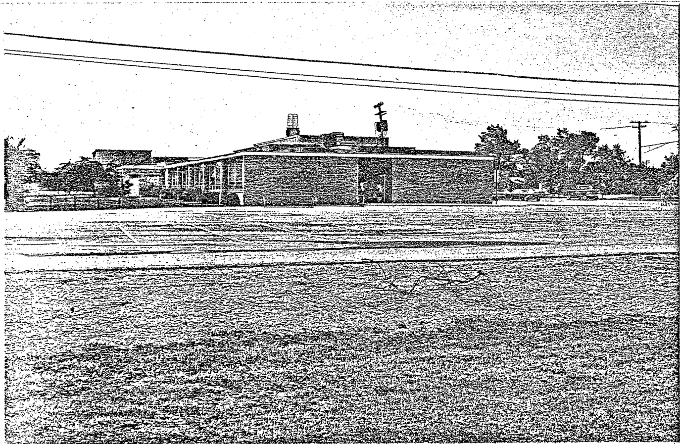
Figure 8. Microphone located 50 ft N of NE corner of Congregation B'nai Moshe on NE corner of Church and 10 Mile Rd, observer looking SW. Sta. 222.
