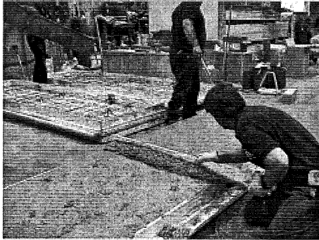
Figure 50. Concrete Surface Finishing.
