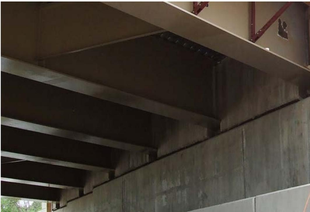
Figure 4.8 The reinforced concrete end diaphragm / back wall of the Woodruff Bridge
