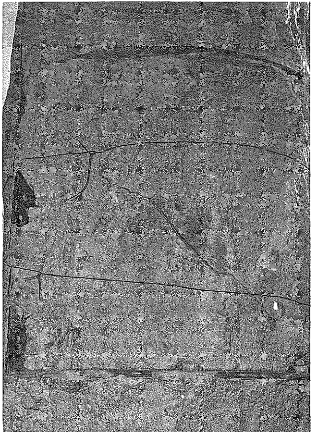
Figure 1. Steel column form (above), with foam applied (top left). Note tie wires (lower left).
