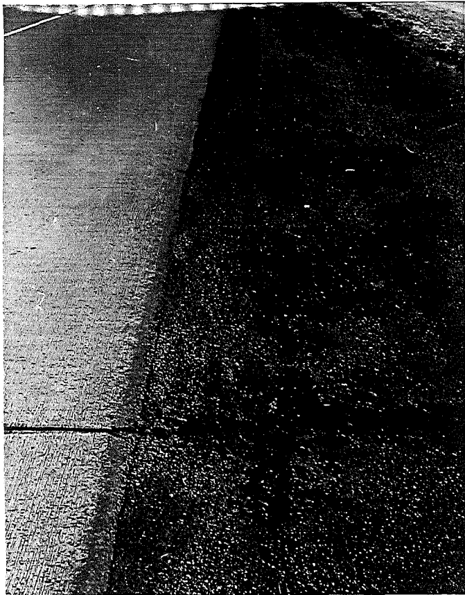
Station 1671+30 -.Inner Shoulder.
