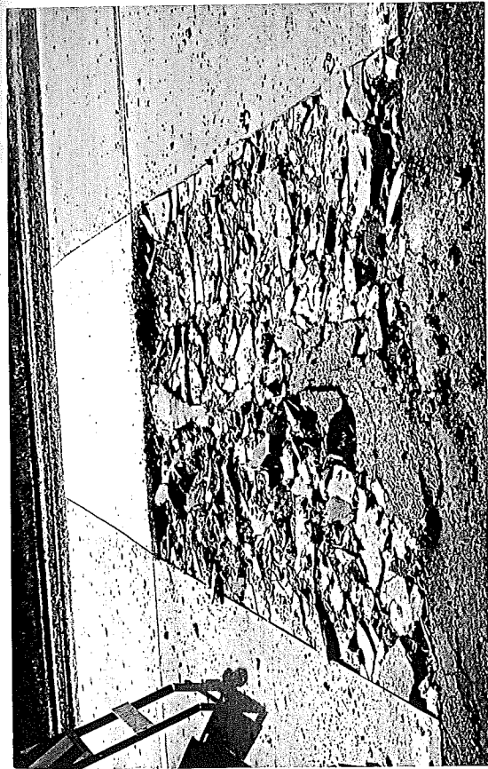
Figure 13. Joint repair in progress. Saw cuts have been made and concrete broken with drop hammer. Project 47-26, C6.
