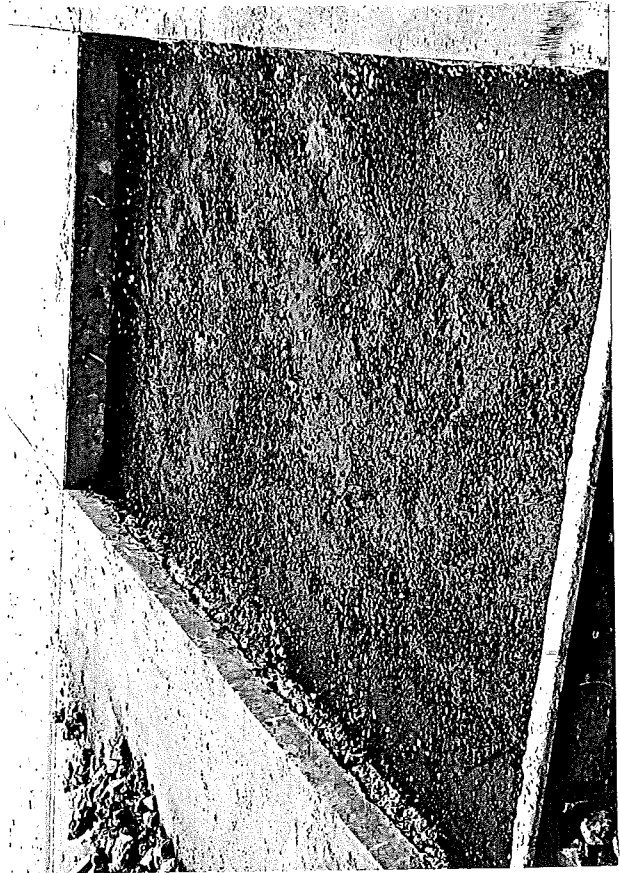
Figure 13. Joint repair in progress. Saw cuts have been made and concrete broken with drop hammer. Project 47-26, C6.
