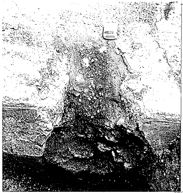
Figure 6. Joint at 316+00. Note deteriorated concrete at bottom of joint. Project 47-26, C6.
