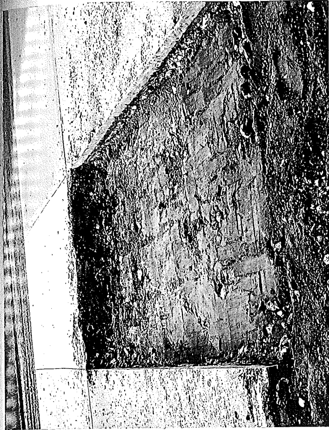
Figure 13. Joint repair in progress. Saw cuts have been made and concrete broken with drop hammer. Project 47-26, C6.
