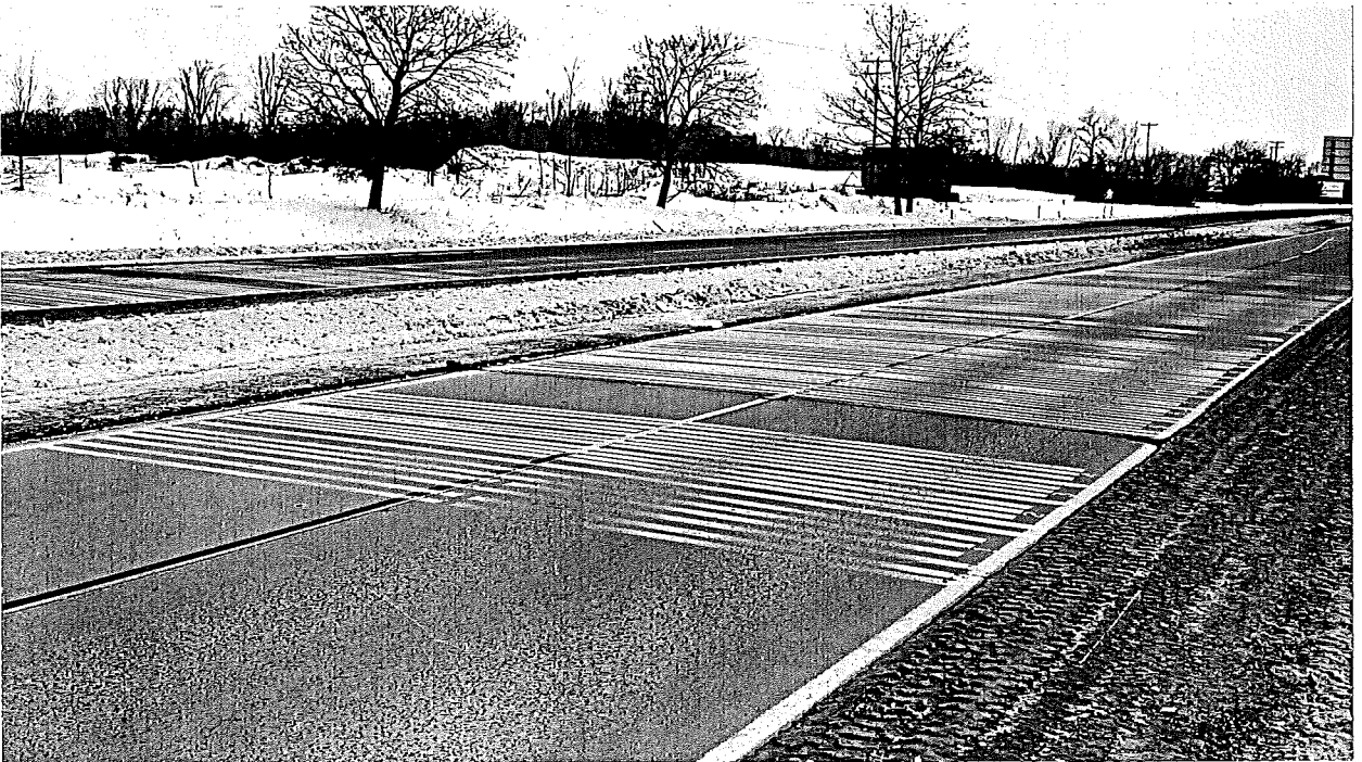
Figure 2. Appearance of test stripes on EB M 78 (Concrete) at time of last rating. Photo on 12/14/72. Incidentally, snows came earlier this year than last.
