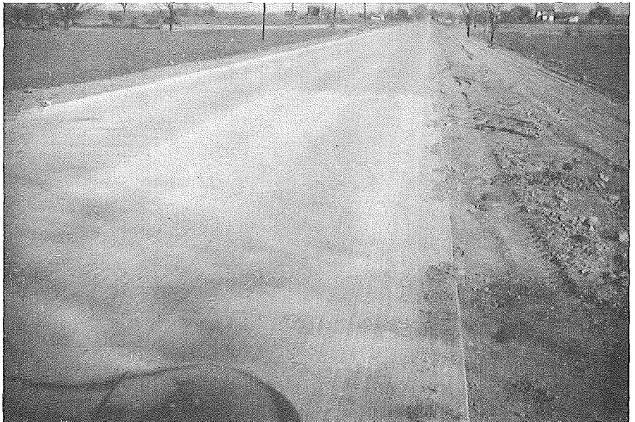
Fig. 20. White membrane 2 months after application.
