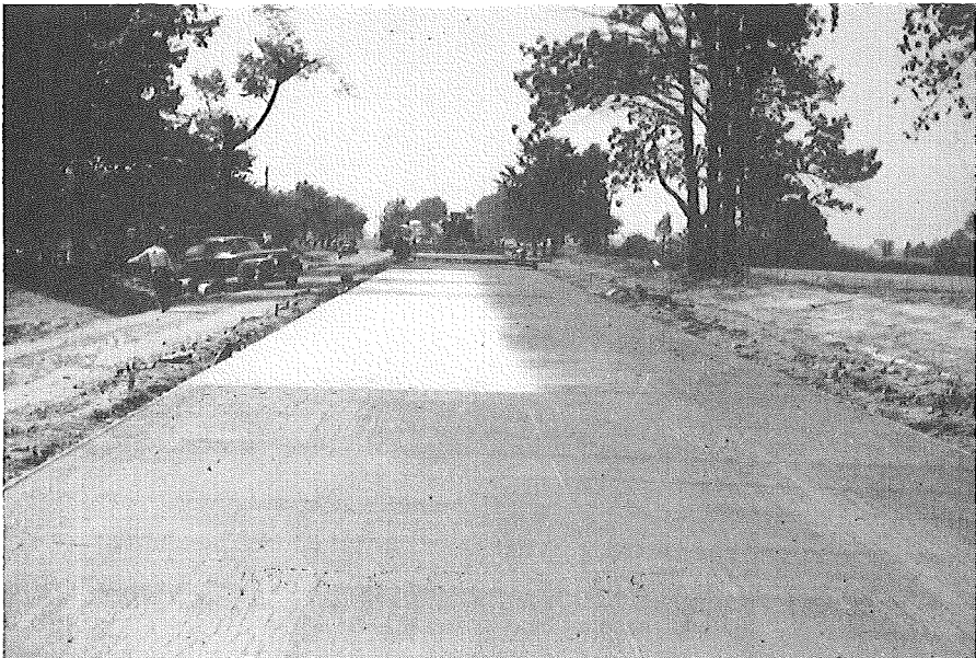
Fig. 18. White membrane immediately after application.
