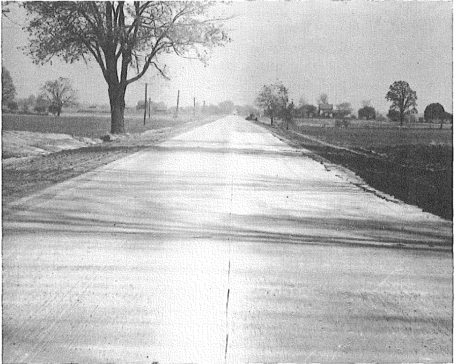
Fig. 19. White membrane one month after application.
