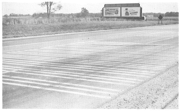
Figure 2. 1957 test stripes in Area 4B were smudged over with asphalt droppings from trucks a few weeks after deposition. Yellow stripes in upper photograph; white stripes in lower photograph.
