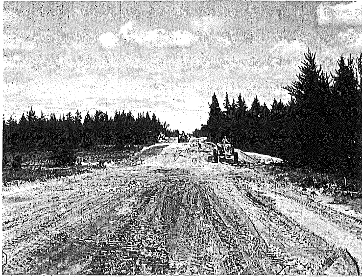
(A) - Grading Operations
