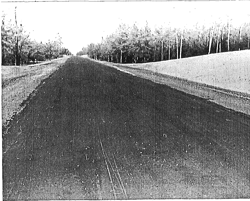
Figure 32. General view of RC-2 section, station 119+00.
