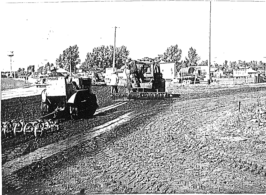
Figure 17. Application of bituminous material
