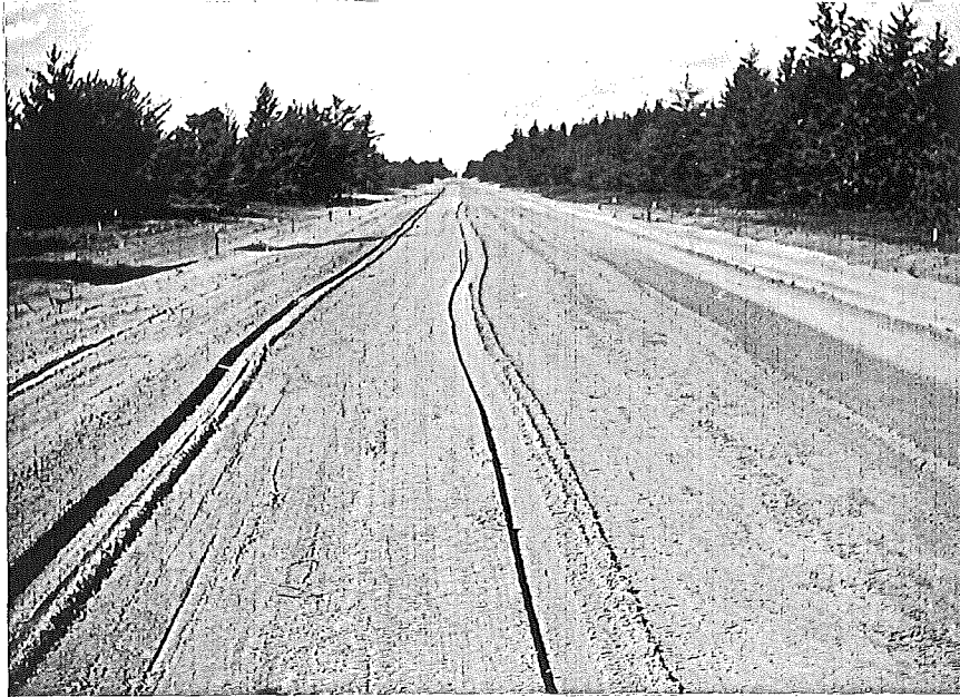
Figure 16. Sand subgrade prior to application of bituminous binder.
