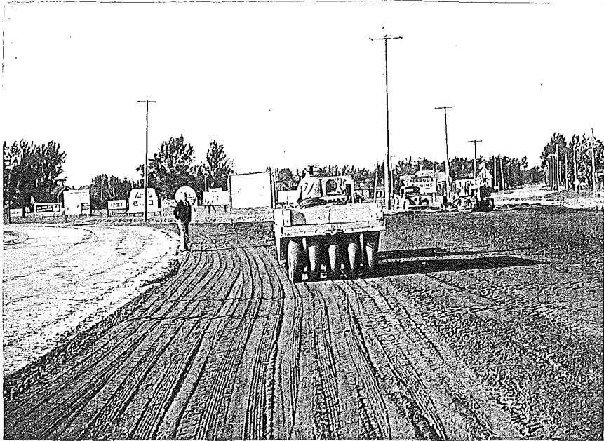
Figure 25. Compaction with rubber tired roller
