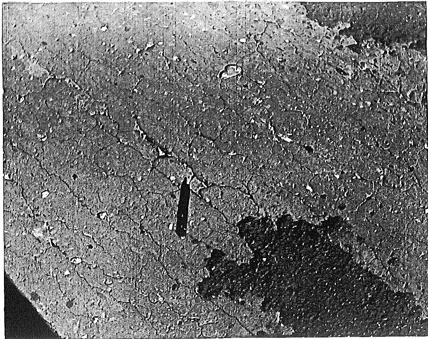
Figure 43. MC-2 section, station 246. Note longitudinal cracking.
