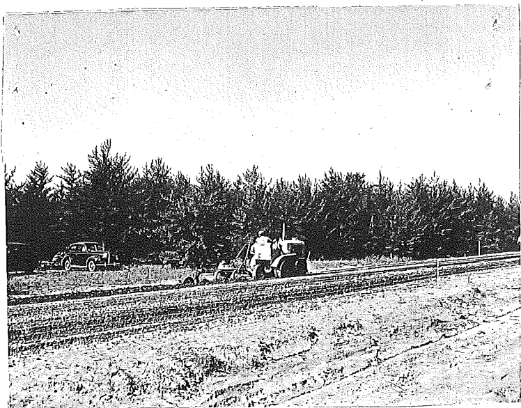
(B) Turning in cement with 3-bottom gang plow
