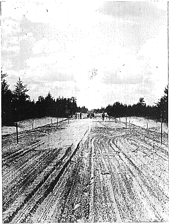
(B) - Spreading Limestone Dust
