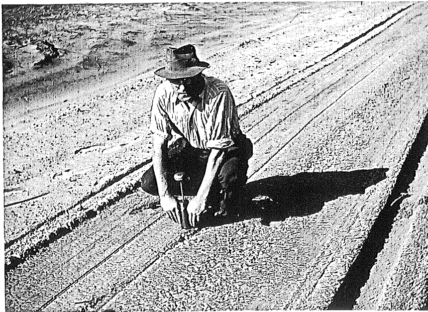
Figure 15. Sampling the subgrade prior to application of bituminous material.
