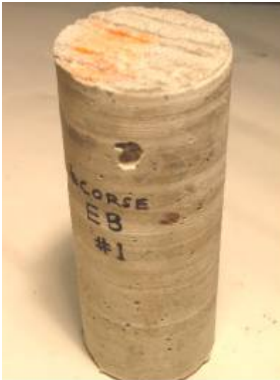
Figure 3.86. Core 5a with a large void
