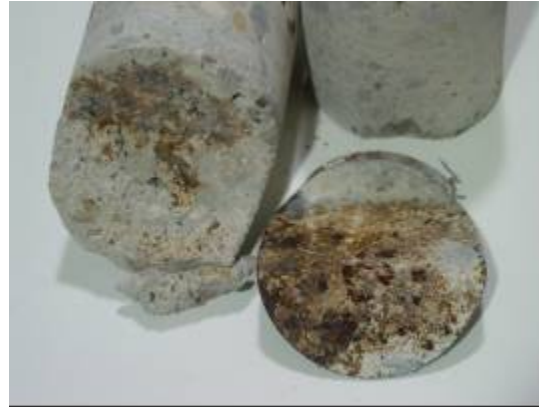
Figure 3.107. Core 6d rust on the SIPMF
