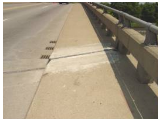
Figure 3.8. Different types of concrete around the joints
