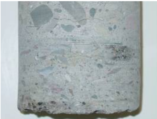
Figure 3.174. Core 10a horizontal crack.
