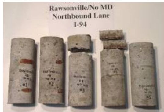
Figure 3.32. The 5 cores taken from Bridge Deck Number 2 (Structure No. S03-81041)
