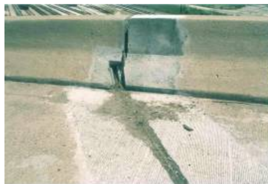
Figure 3.165. Different types of concrete around the joints
