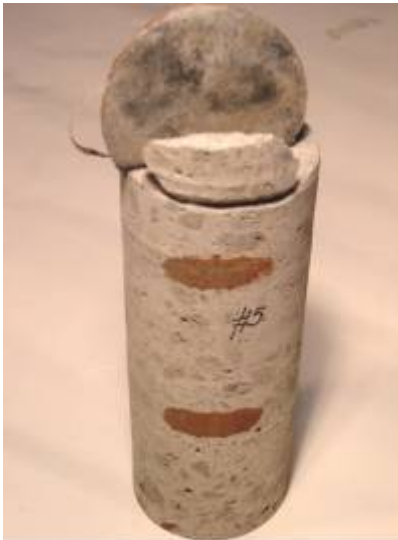
Figure 3.122. Broken concrete in the region of the valley of the SIPMF and the rust in the reinforcement bars in Core 7e
