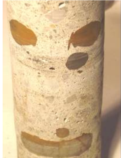
c. Rusted reinforcement bars
