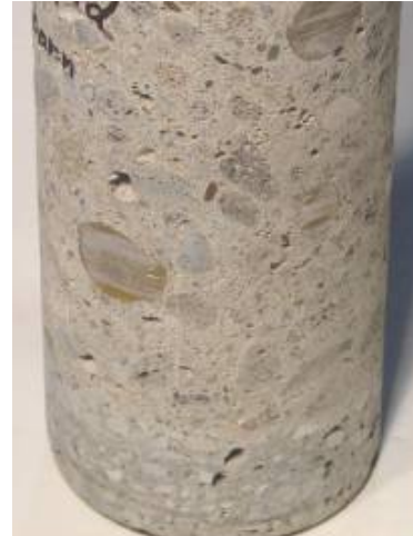
b. Entrapped air voids in the wearing surface
