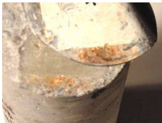
Figure 3.153. Core 9d rust traces on SIPMF and concrete
