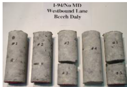
Figure 3.72. The 5 cores that were taken from Bridge Deck Number 4 (Structure No. S11-82022)
