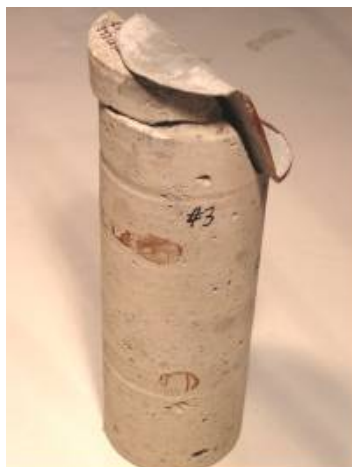
Figure 3.120. Core 7c shows the broken concrete in the region of the valley of the SIPMF and the rust in the reinforcement bars
