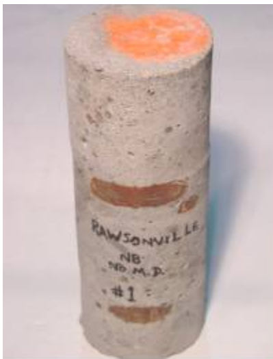
Figure 3.33. Core 2a reinforcement bars are rusted
