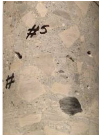
Figure 3.78. Voids observed in Core 4e
