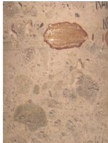
b. Rust in the reinforcement bar
