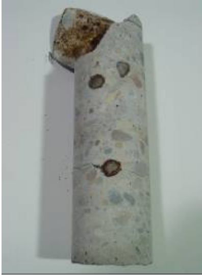
Figure 3.105. Core 6c crack at the reinforcement
