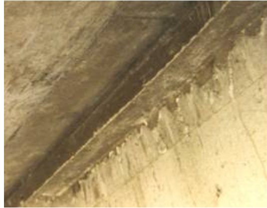
Figure 3.71. Good concrete condition
