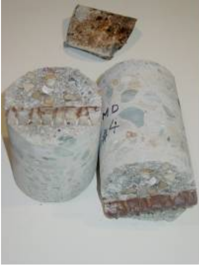
Figure 3.106. Core 6d rust at the reinforcement bar
