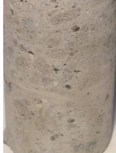
b. Large voids
