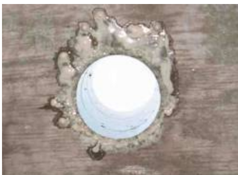
d. Resulting hole in a concrete deck slab without SIPMF, view from below
