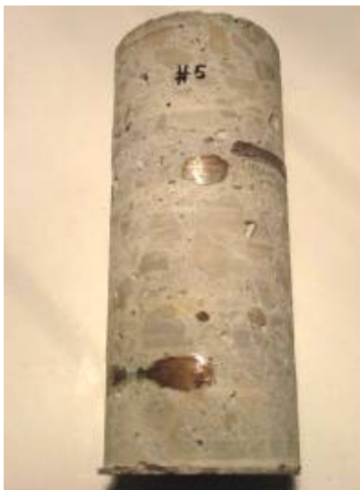
Figure 3.91. Core 5e with rust traces in reinforcement bars
