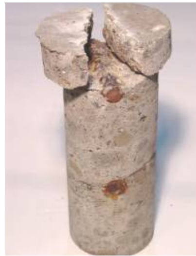
b. Reinforcement bars are rusted
