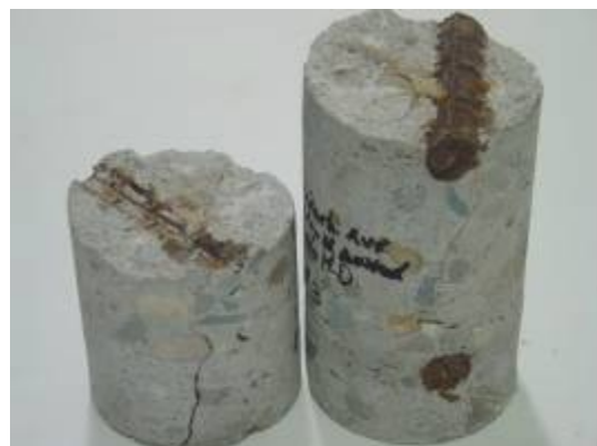
Figure 3.15. Core 1c rust in steel
