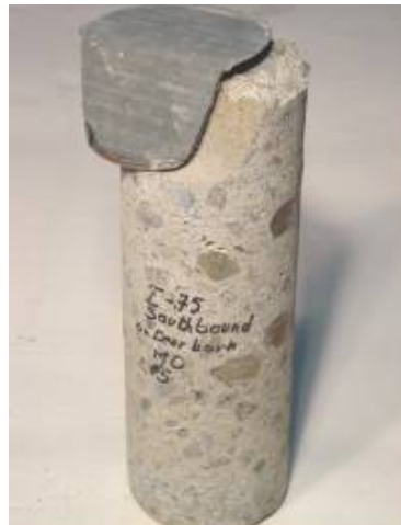
Figure 3.137. Core 8e with the broken concrete in the region of the valley of the SIPMF
