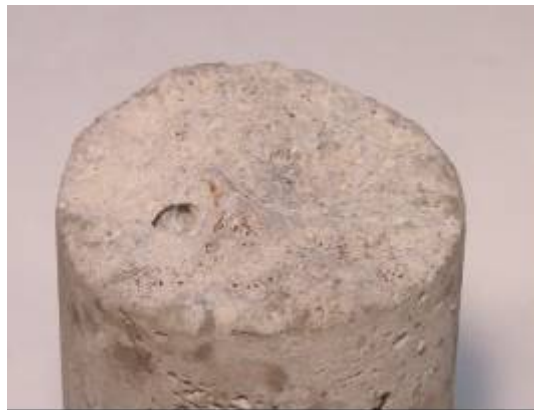
Figure 3.41. Core 2c honeycombing in the concrete
