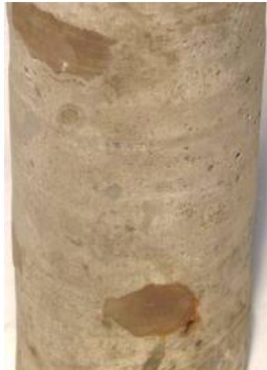
Figure 3.65. Rust in steel bars Core 3e
