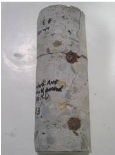
Figure 3.14. Core 1c transverse and longitudinal cracks
