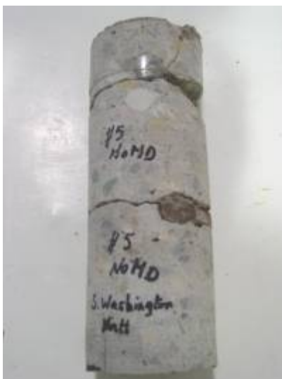
Figure 3.17. Core 1e cracks at the reinforcement bars
