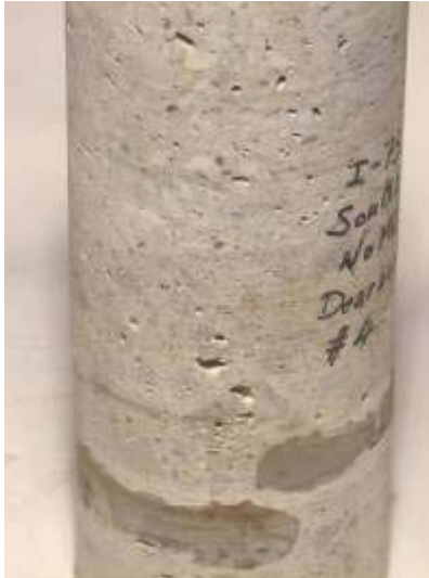
Figure 3.63. Voids in Core 3d
