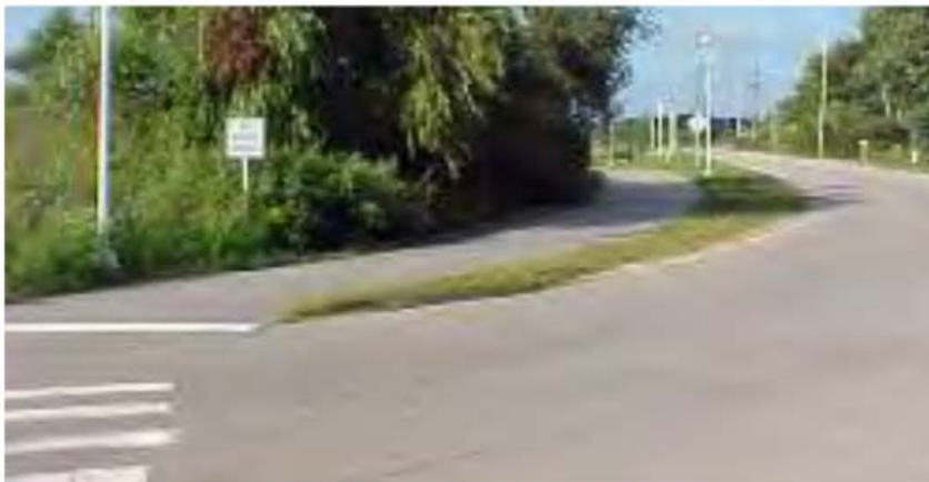
Sidepath (Michigan Department of Transportation 2014a)
