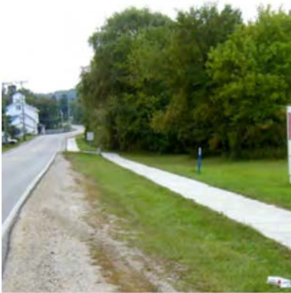
Sidewalk (Michigan Department of Transportation 2014a)
