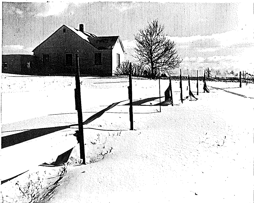
Figure 8. Another view of 2-panel fence on east side of US-131 N. of Cadillac, showing damage caused by children. Wexford County, 1-29-52
