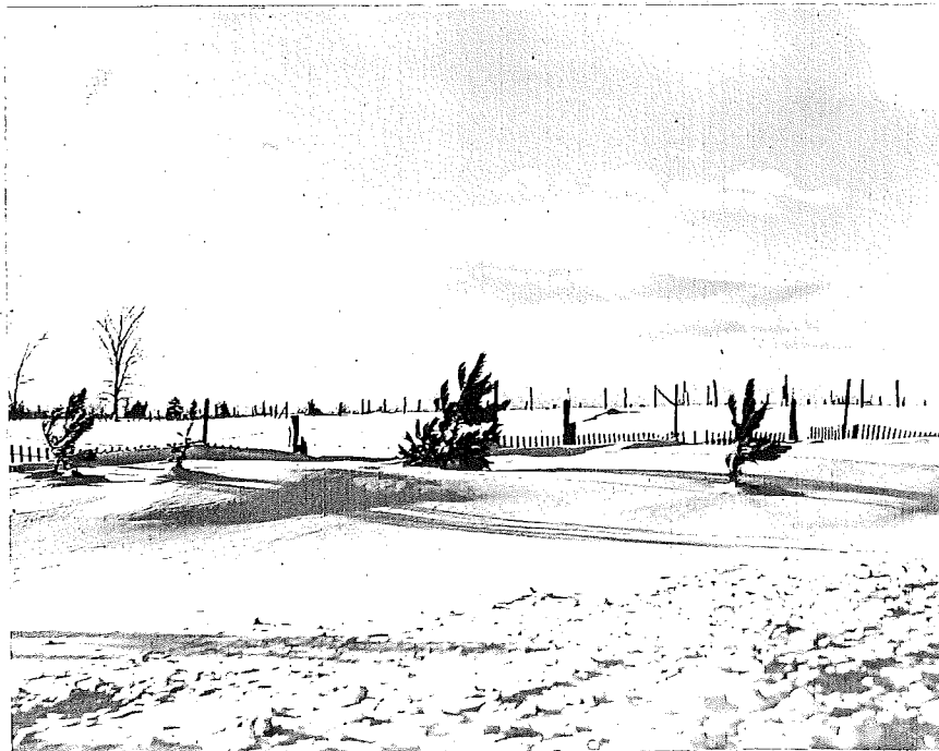
Figure 15. Picket fence that has stopped functioning, along US-131 N. of Cadillac. Wexford County, 1-29-52
