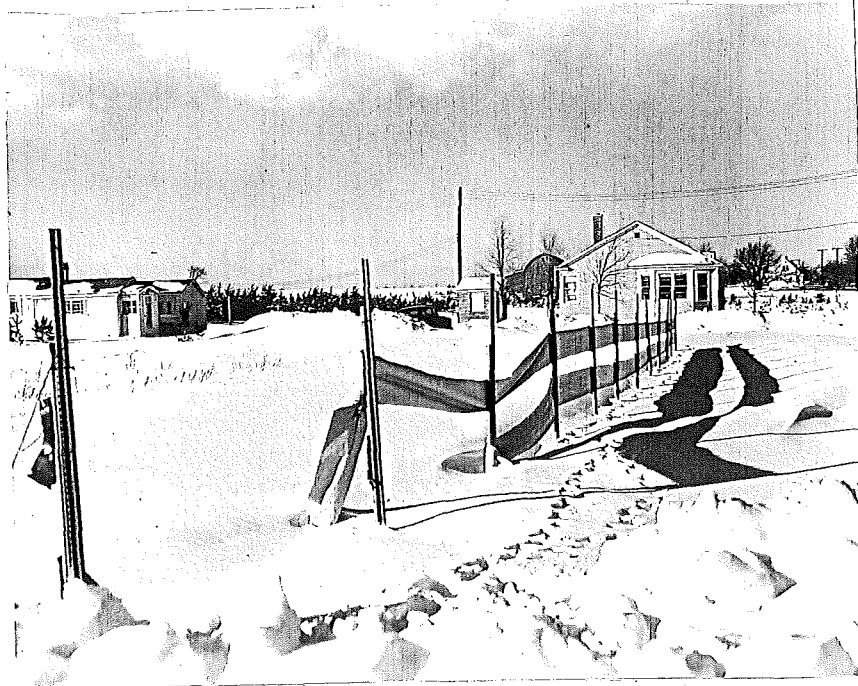
Figure 12. 2-panel fence on west side of US-131 N. of Cadillac; reported broken by children. Wexford County, 1-29-52
