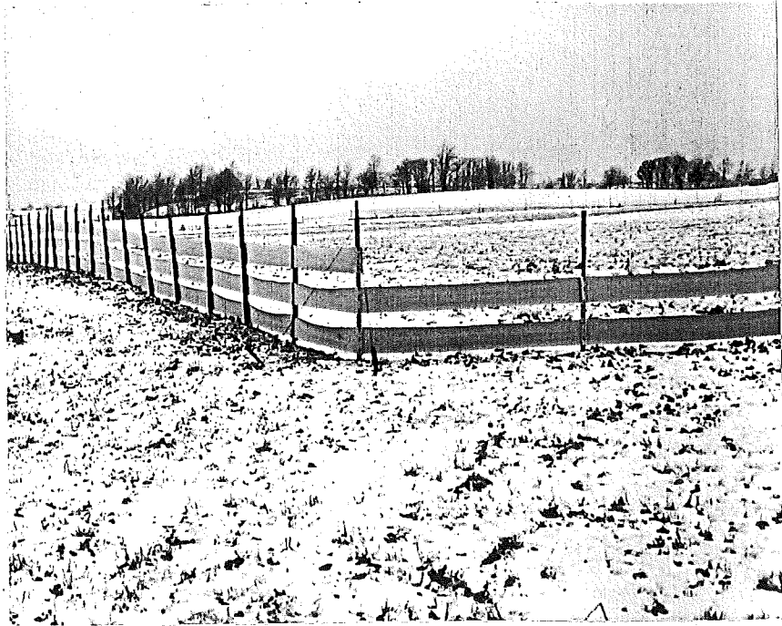
Figure 30. 2- and 3-panel stretch of fence on north side of US-12 in Jackson County east of Ludlow Road, showing method of taking fence around corners. 2-7-52
