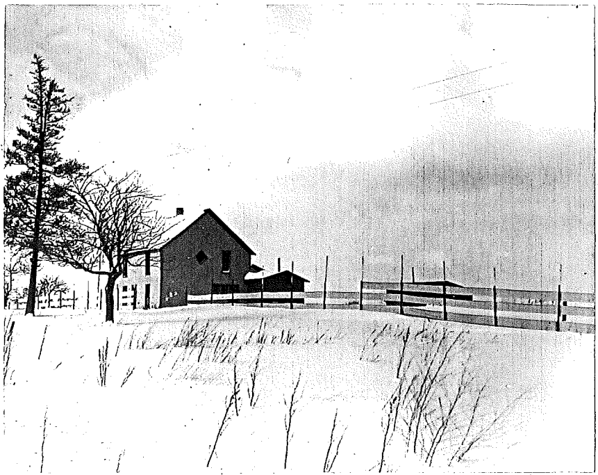
Figure 3. On north side of M-144 N.E. of Roscommon - 2- and 3-panel fence with provision for raising. Roscommon 1-29-52
