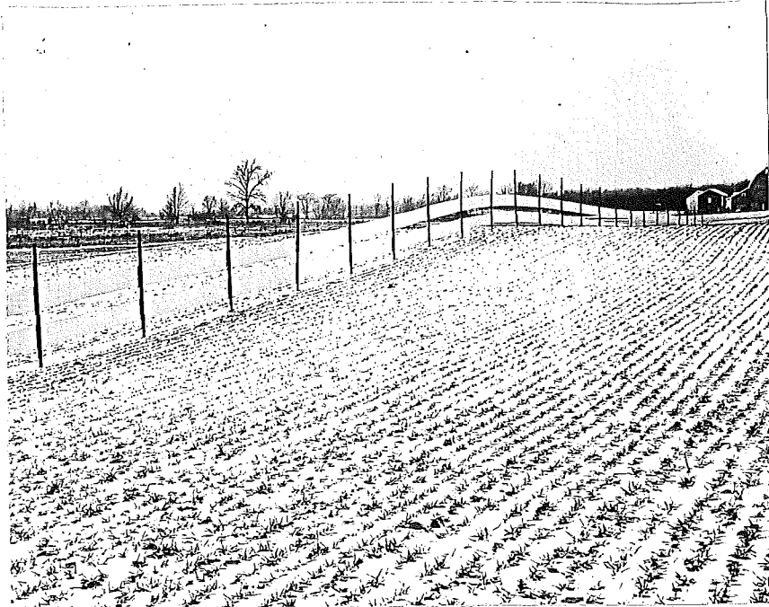
Figure 26. North section of 2-panel fence on west side of US-127 in Jackson County just south of Ingham County line, showing installation in rolling topography. 2-7-52
